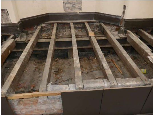
Floor boards removed and steel frame base uncovered and surveyed
