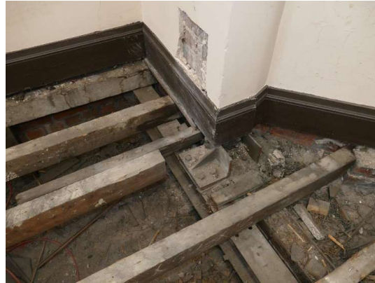
Internal beams supporting the previous remedial support frame and the original construction
