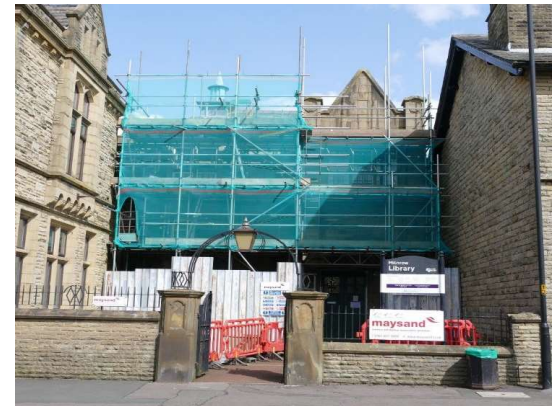
Scaffolding to the front of the building.
