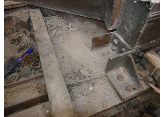
Steelwork added around 2000 to give additional support to the window
