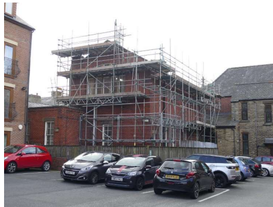
Scaffolding to the rear and side of the building
