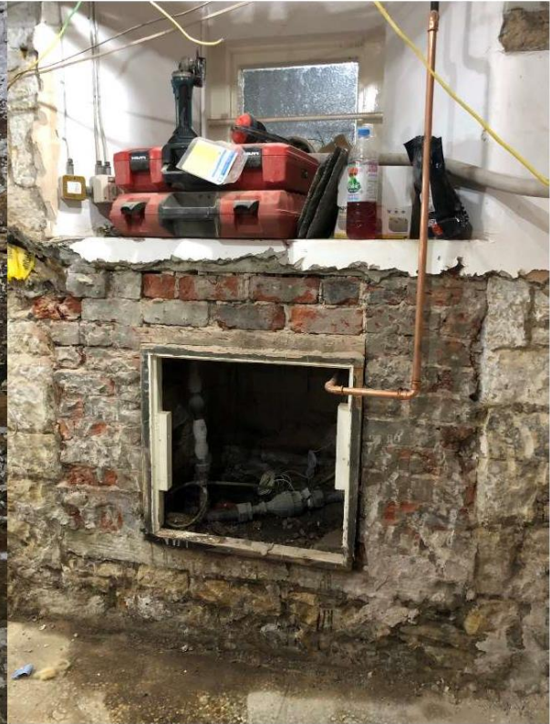
Window infill to be removed (view from B7f).
