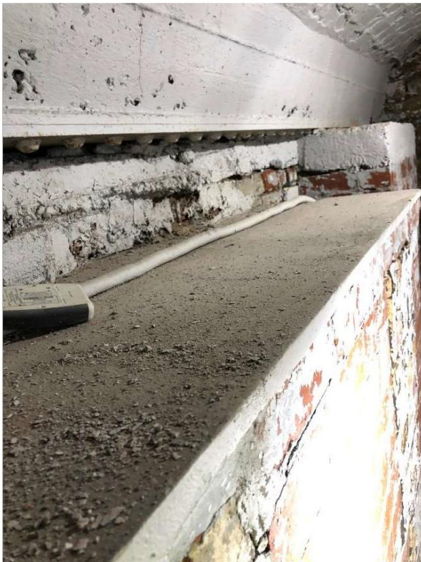
Chimney breast previously capped off.
