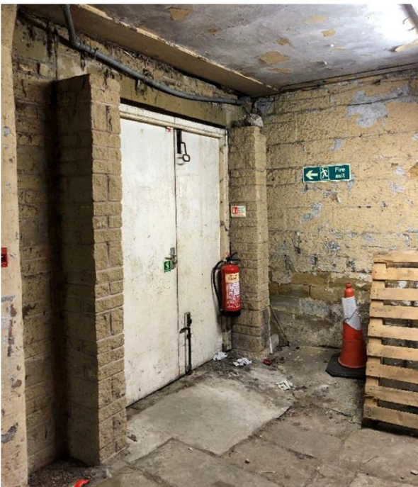
External walls to be dismantled in B7a.
