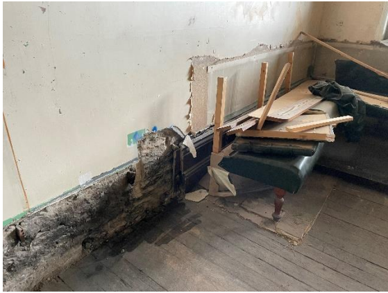
Item 2.9 - Removal of 1990s bar benching.
