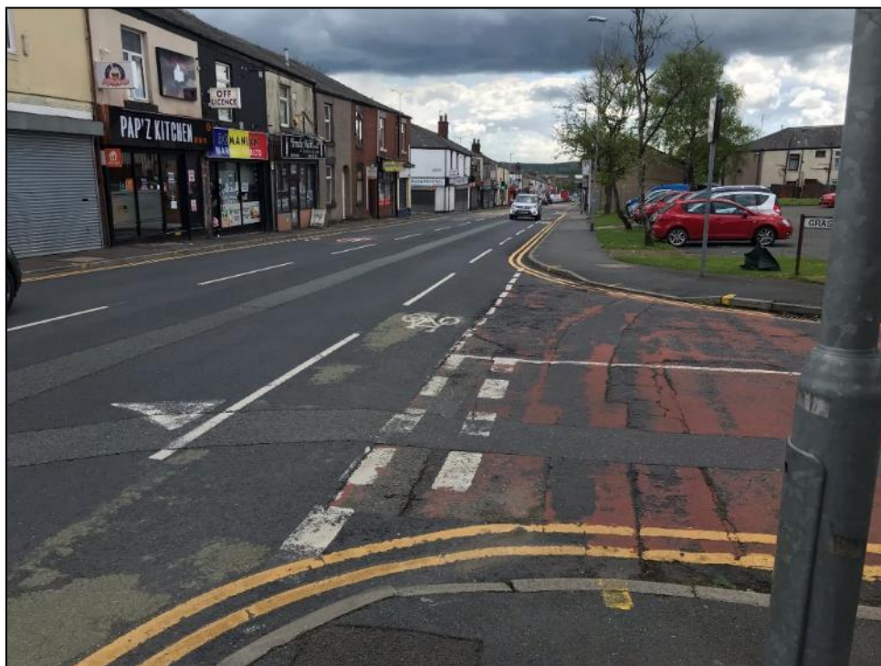
Figure 2. A671 Whitworth Road in vicinity of site
