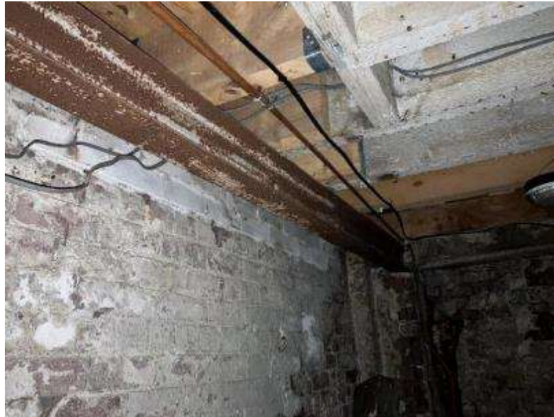
Figure 11 – Steel Beam Supporting Joist Ends
