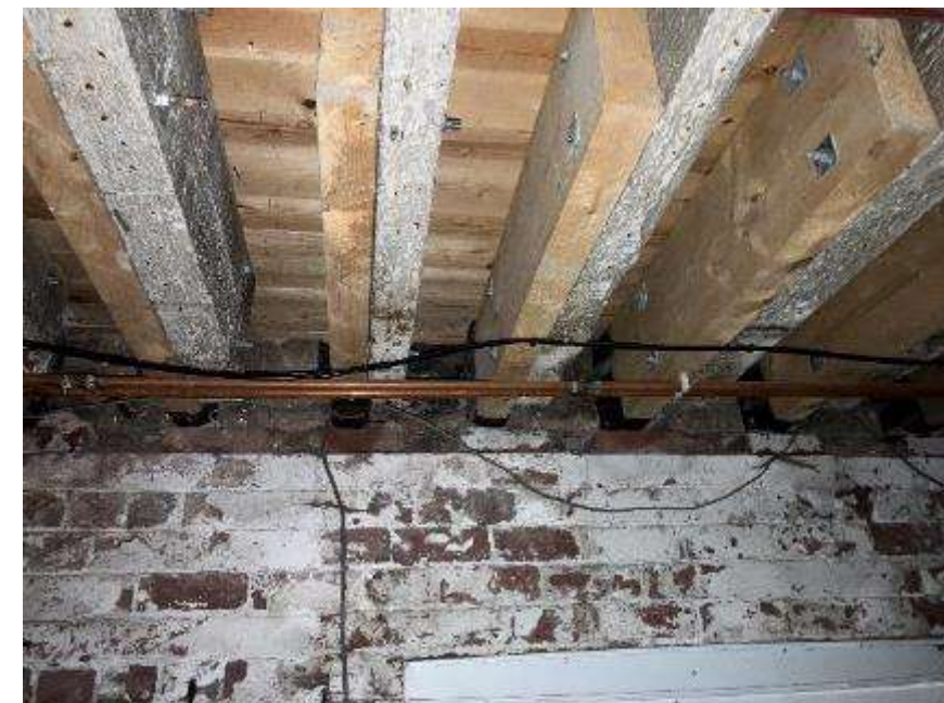
Figure 10 – Historic Timber Repairs to South Gable Wall
