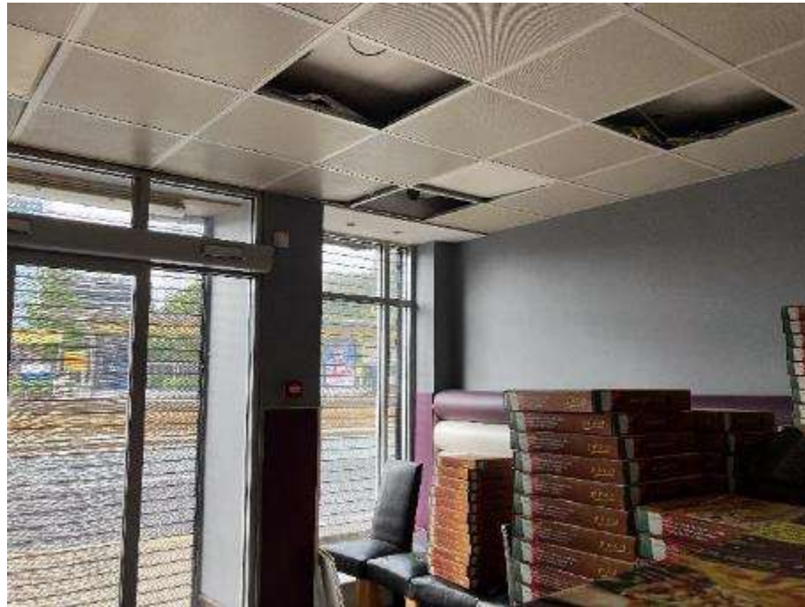
Figure 14 – View on Front Entrance to Kitchen Area
