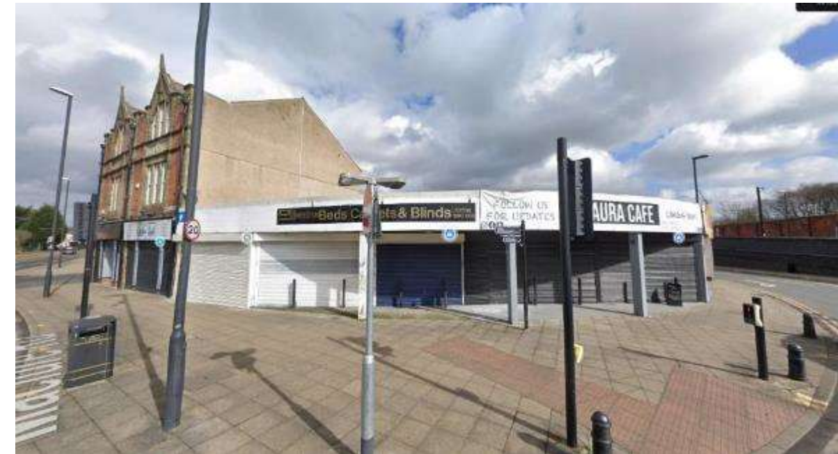
Figure 2 – View on Existing Buildings (Looking North)
