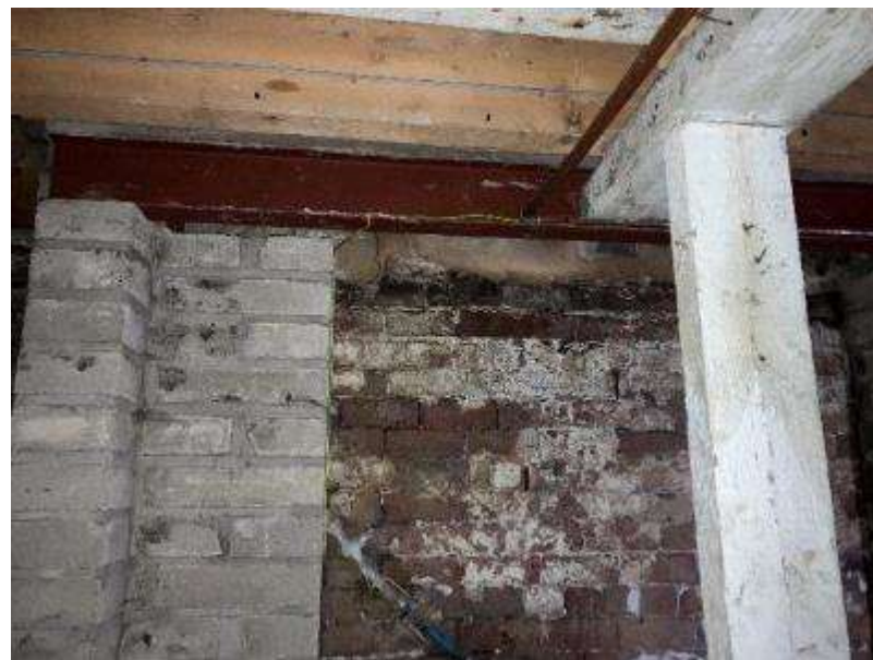
Figure 12 – Steel Support Under Main Entrance Above
