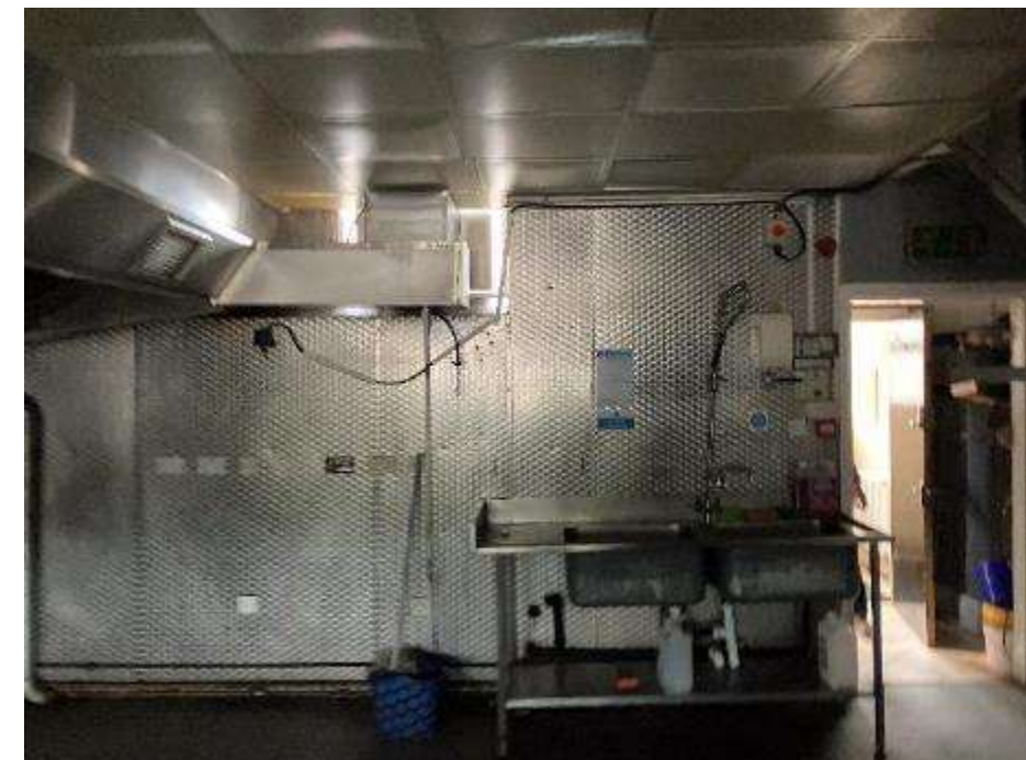
Figure 13 – View on Rear Wall of Existing Kitchen Area
