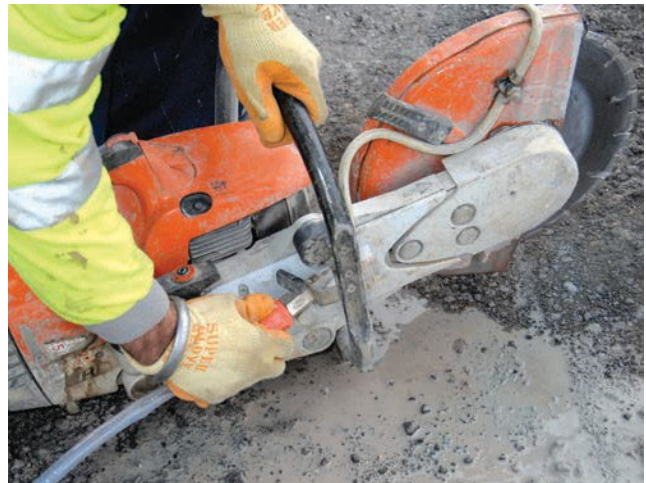
Figure 3 Water suppression on a cut-off saw
