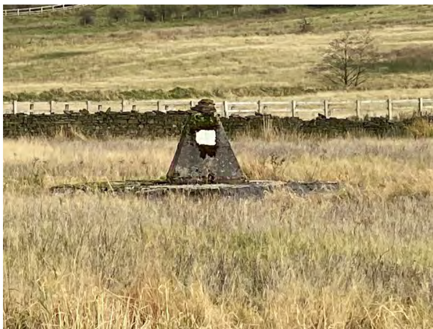
Photo 9) Capped shaft in Northeast adjacent field
