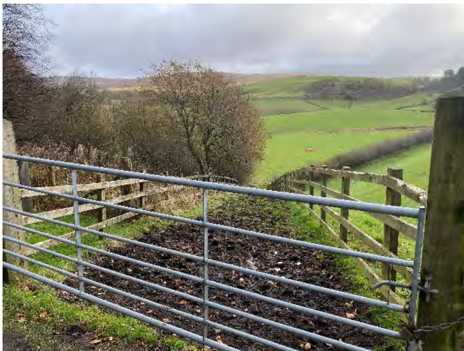
Photo 1) Site Access Looking East. Reservoir embankment on right.
