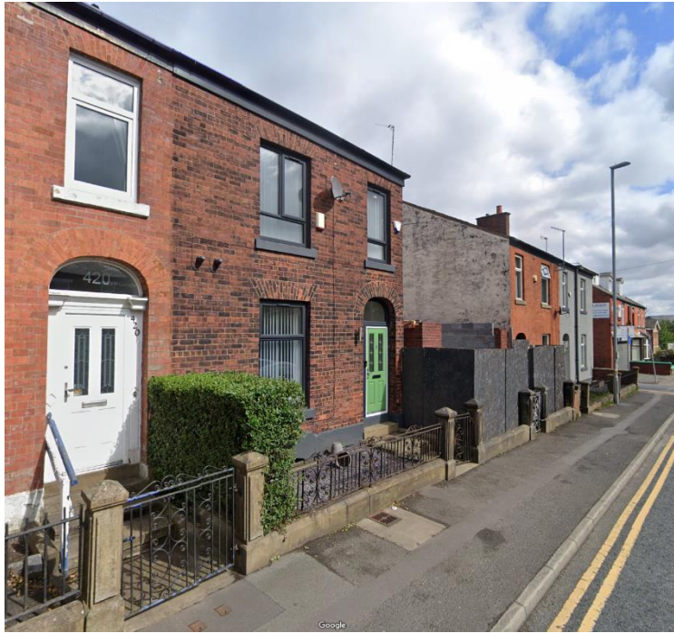
Above: Front elevation of application property.
