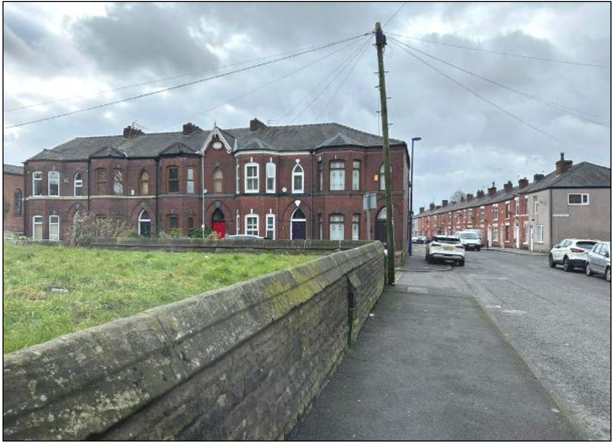
5. Late 19 th century houses on St James' Terrace, and workers' houses on Tower Street beyond
