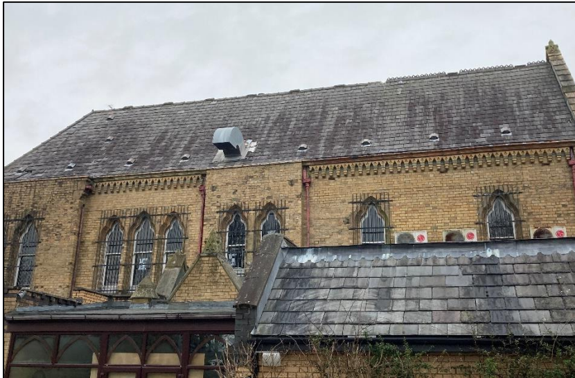
Photograph 17 showing one of the extensions
