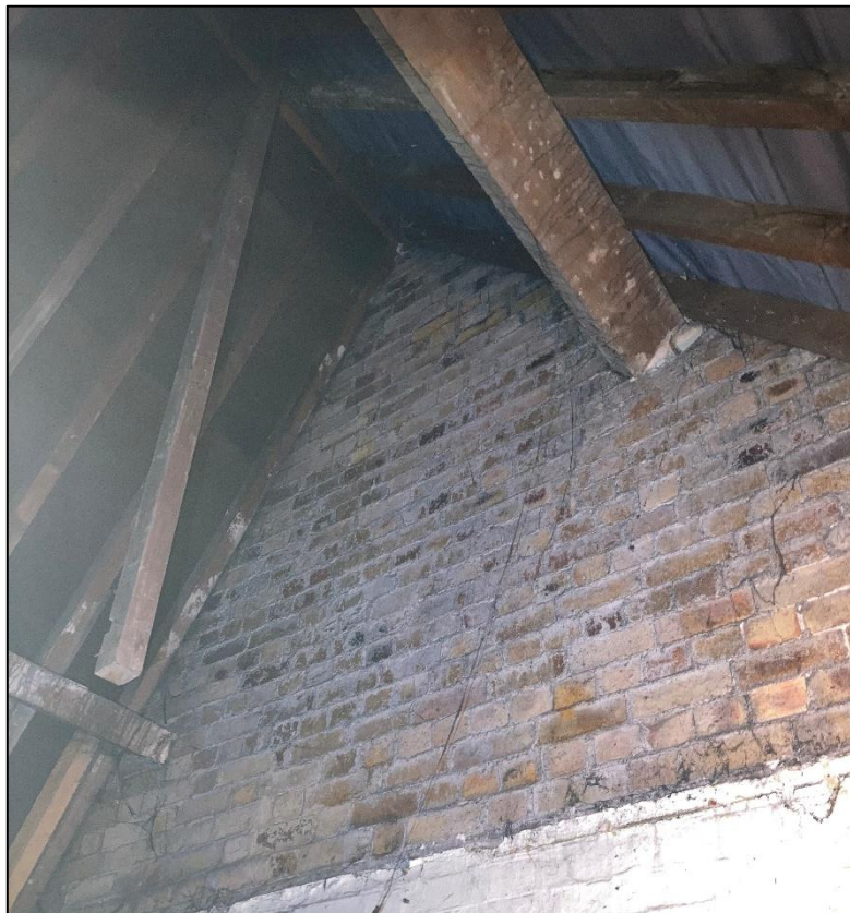
Photograph 29 showing the internal brickwork
