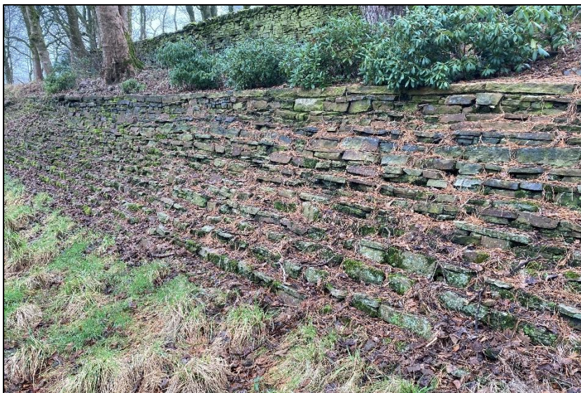
Photograph 13 showing a drystone embankment
