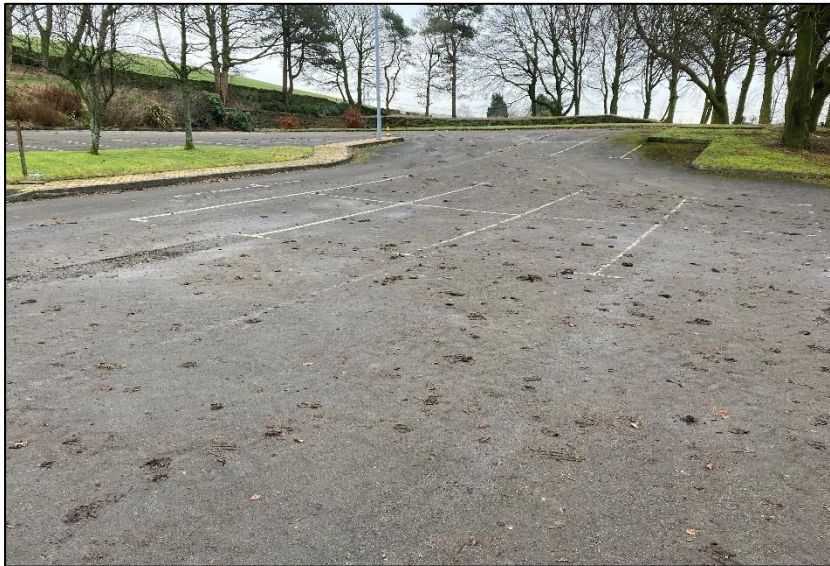
Photograph 1 showing the car park
