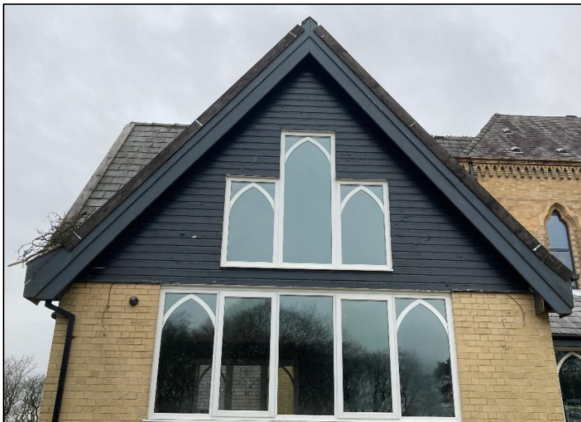
Photograph 16 showing the wooden cladding
