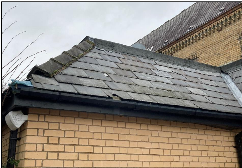
Photograph 20 showing the ridge tiles
