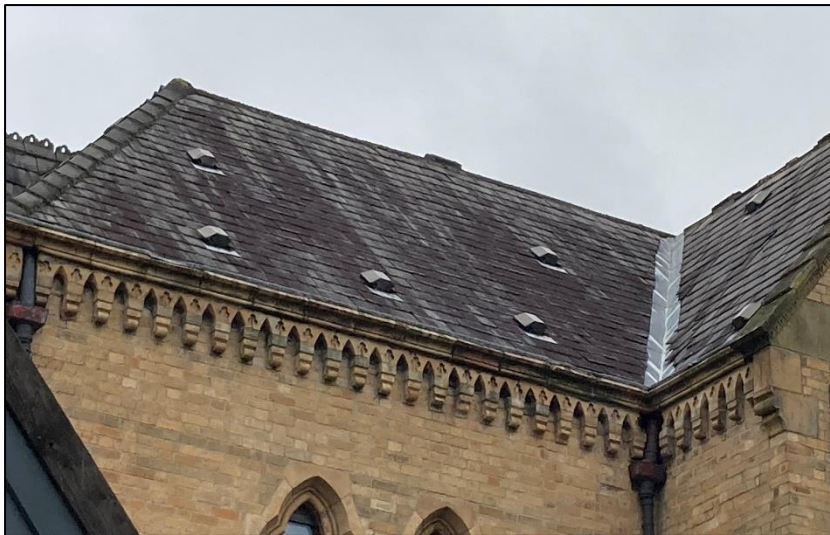
Photograph 21 showing the roof edges
