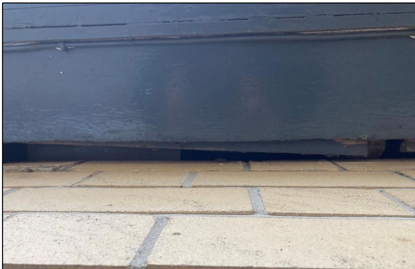
Photograph 22 showing the fascia and soffits
