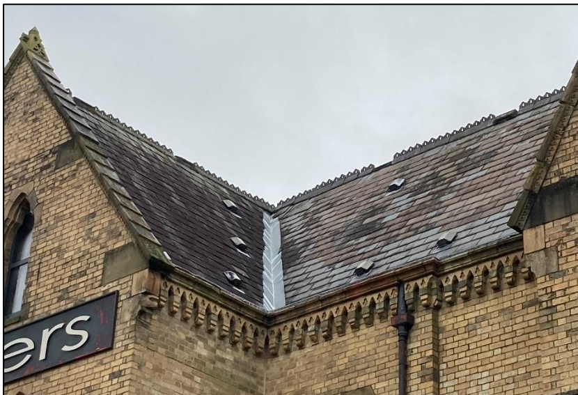
Photograph 18 showing the roof
