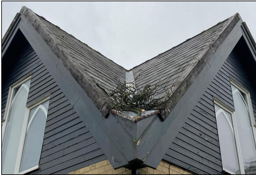
Photograph 19 showing the roof valleys
