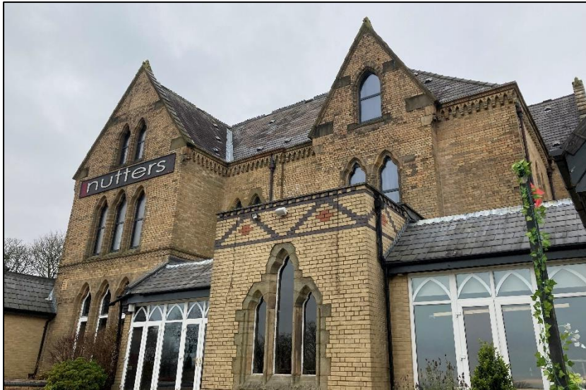
Photograph 15 showing the windows
