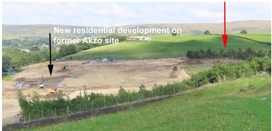
Figure 6 – view from west towards site (red arrow) and AKZO development site now under construction
