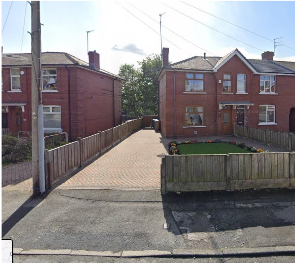
Above: Front elevation of application property.
