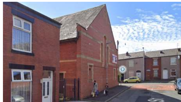
View of site from Medley Street.
