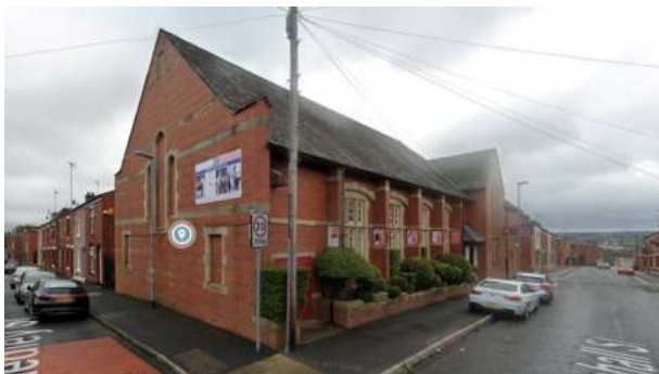
View of site from the corner of Whitehall Street and Medley Street.
