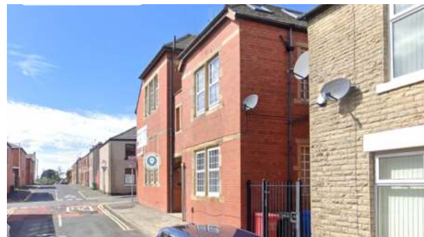
View of site entrance from Milford Street.
