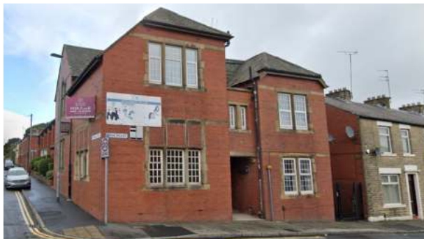
View of site entrance from the corner of Whitehall Street and Milford Street.
