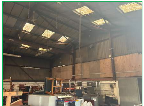
The internal space of Structure B
