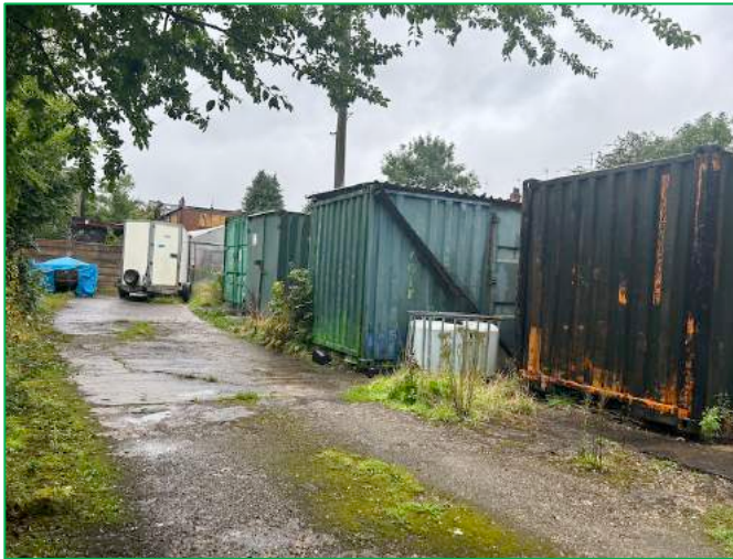
The southwest elevations of the shipping containers
