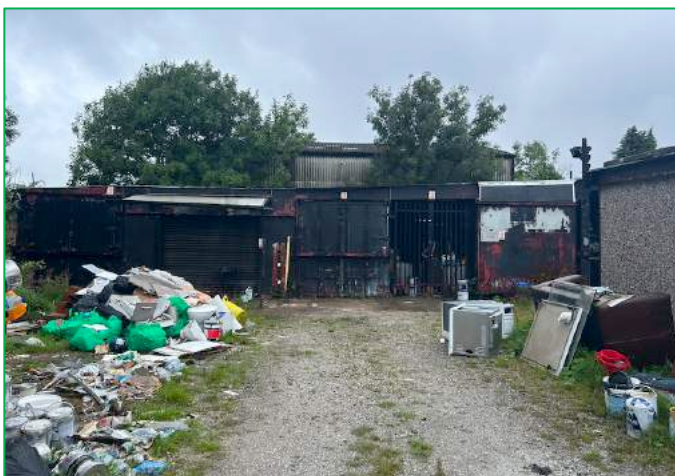
The southeast elevation of Structure C
