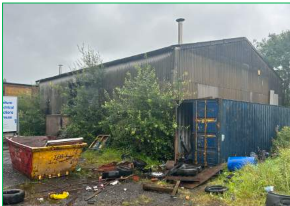
The northwest and southwest elevation of Structure B
