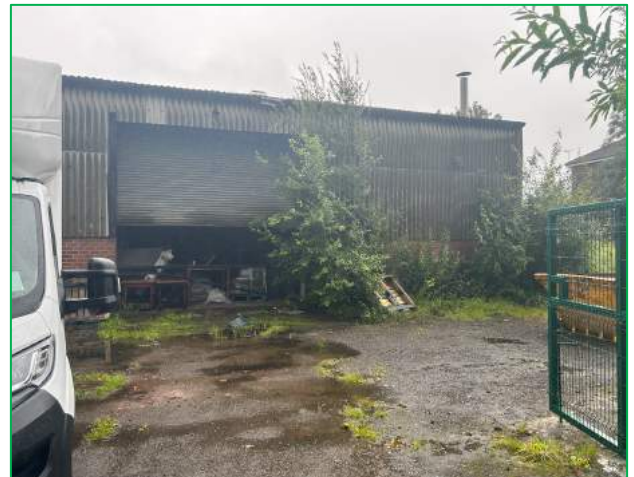
The northwest elevation of Structure B
