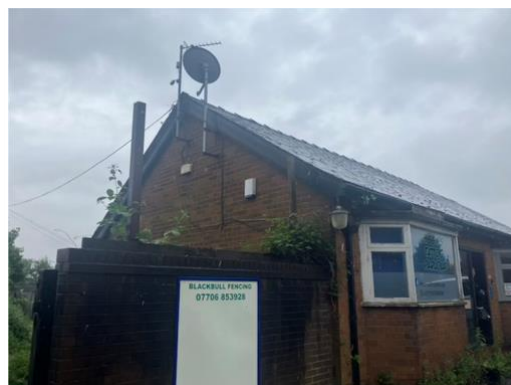
Photo 4: external view of building 1, showing intact slate roof and brickwork.
