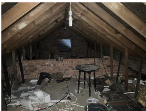
Photo 5: internal view of boarded loft space being used for storage. Roof lining membrane was intact.
