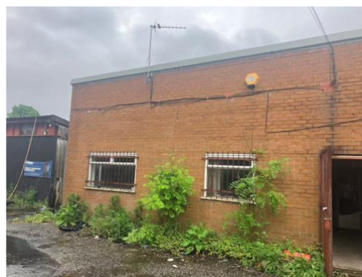
Photo 6: External view building 2.
