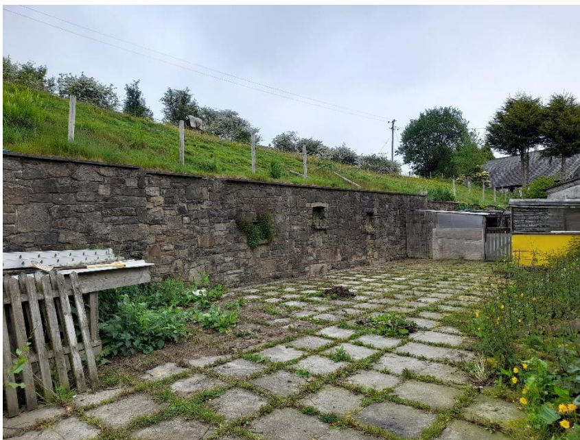
Figure 8 – View to the rear of the property showing the retaining wall to the embankment.
