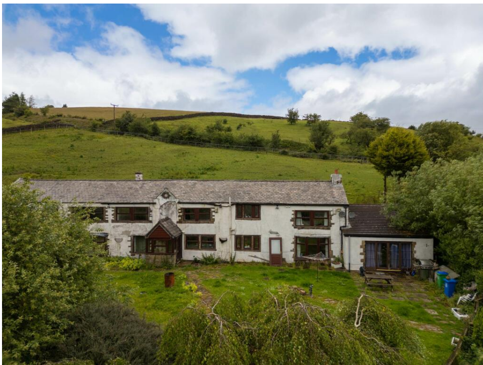
Figure 6 – View of the front elevation showing the split in volumes between the single and 2 storey elements.
