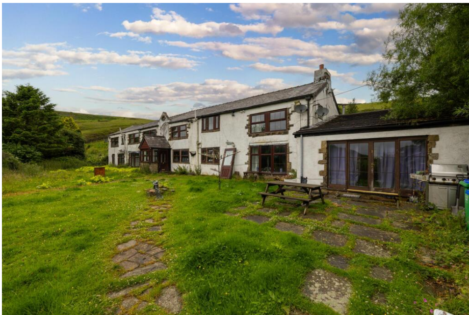
Figure 4 – View of Slack Farm front elevation showing the current residential split.
