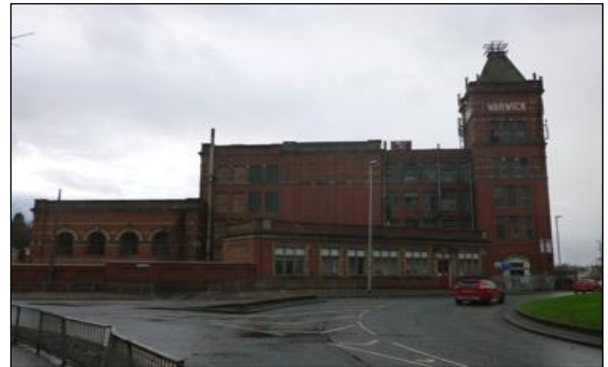
Fig 1 Warwick Mill, Oldham Road view
