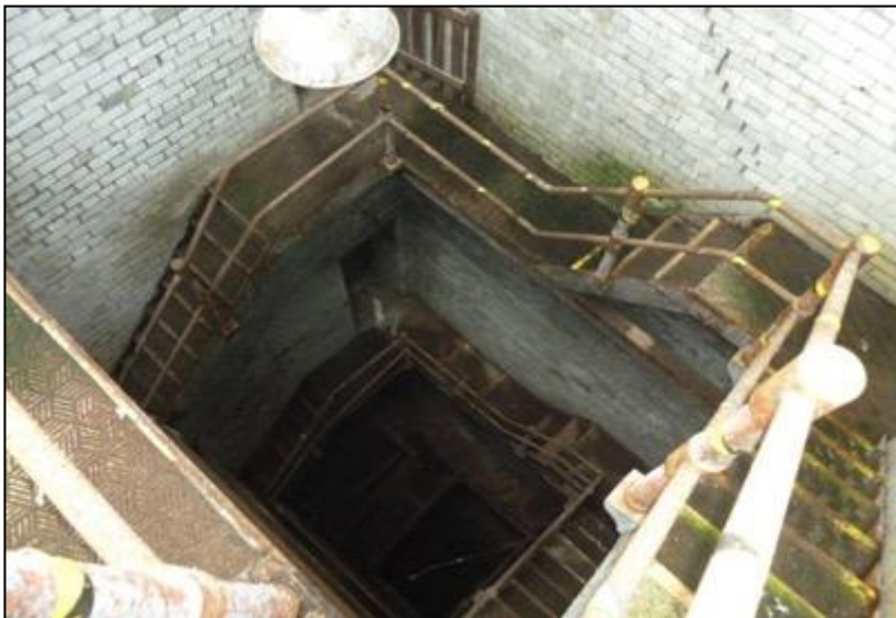
Fig 10 (above) & Fig 11 (below) Rope race Iron staircase
