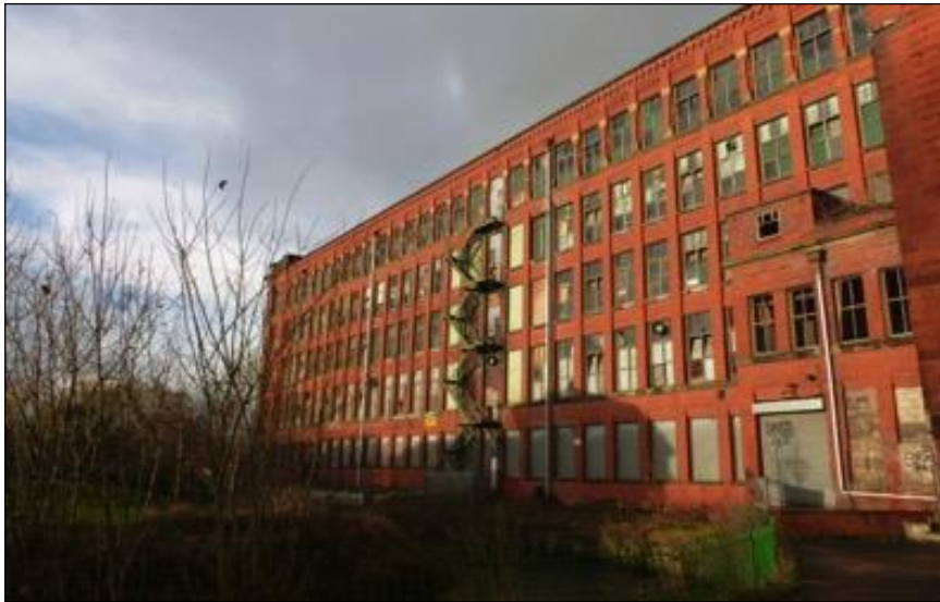
Fig 6 Warwick Mill, Southern Elevation
