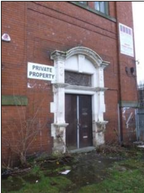
Fig 8 Entrance to stair tower
