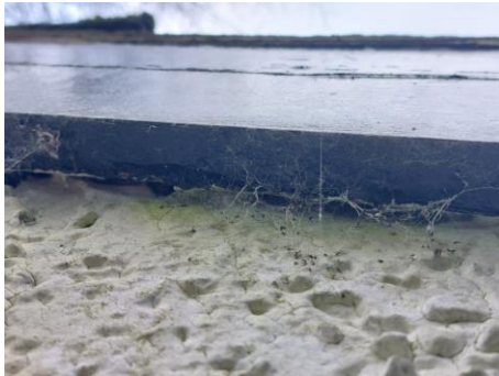
Plate 4: Typical view of fascia underside, close view with no PRF and cobwebs.
