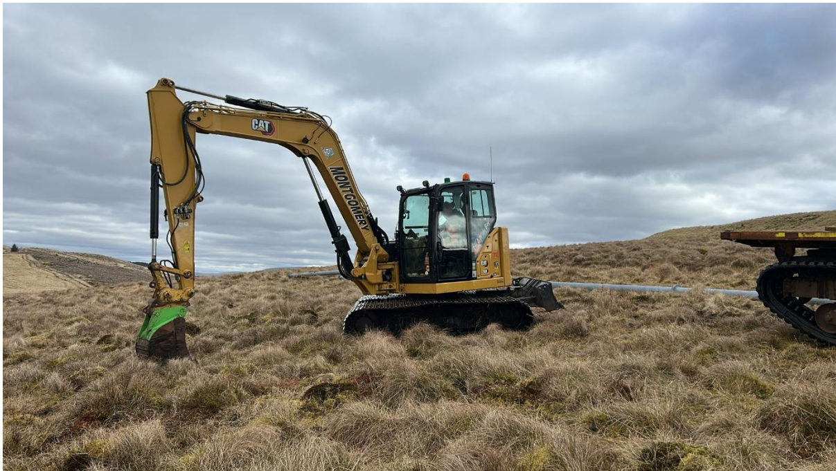
Tracked excavator (8T)
