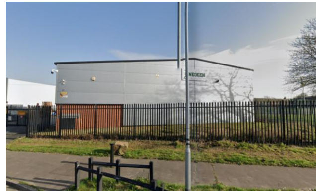
Existing NeoGen Main Facility
