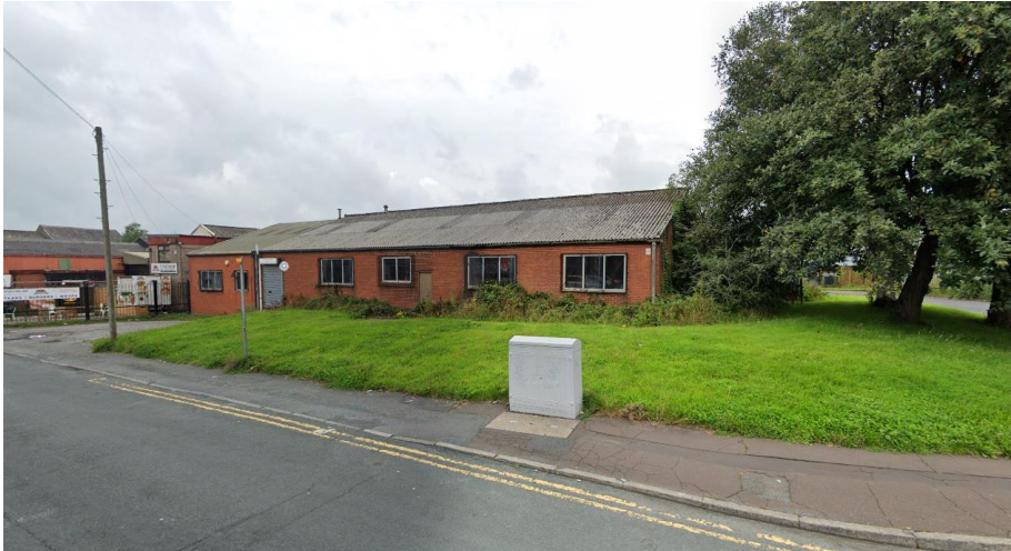
Existing Site Street Scene
