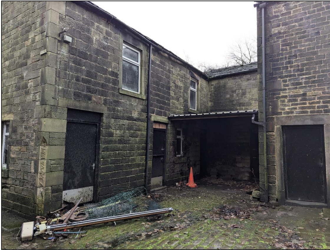
Plate 17: Rear elevation of stable block
