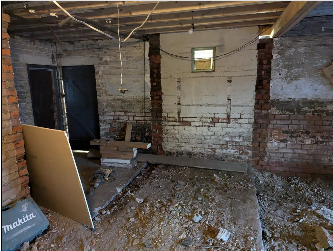
Plate 37: Inserted wall showing scars of removed walls
