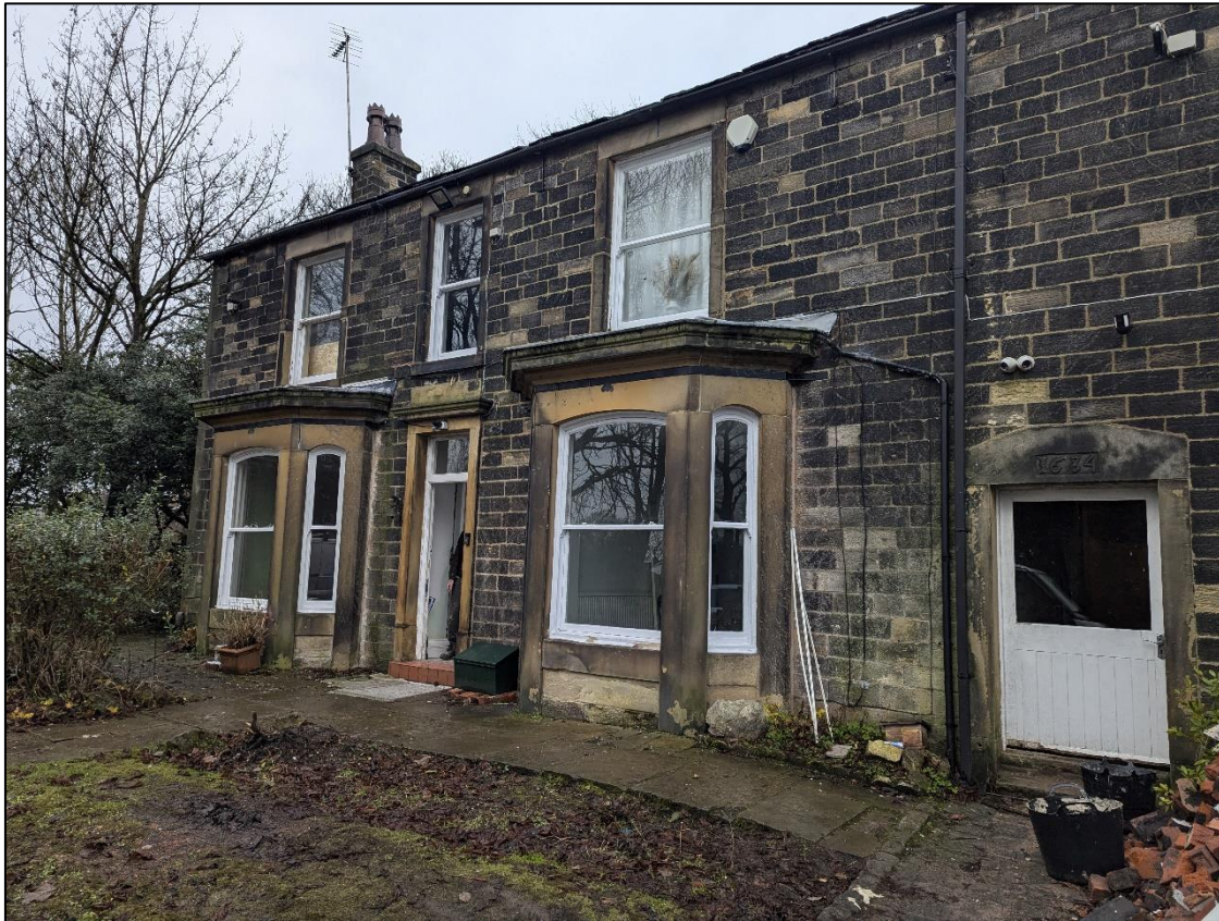
Plate 3: South elevation of house
