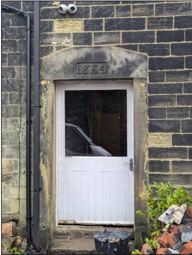
Plate 9: Western doorway with reused lintel bearing date 1684
