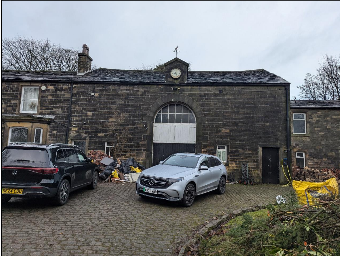
Plate 6: South elevation of barn
