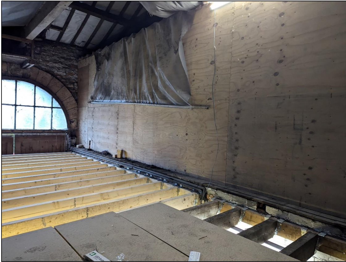
Plate 49: Inserted ply wall to western bay
