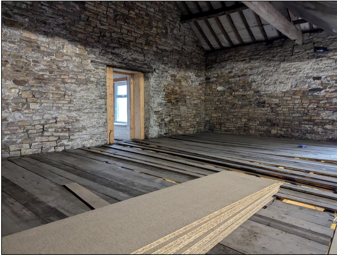
Plate 47: Inserted doorway to stable block
