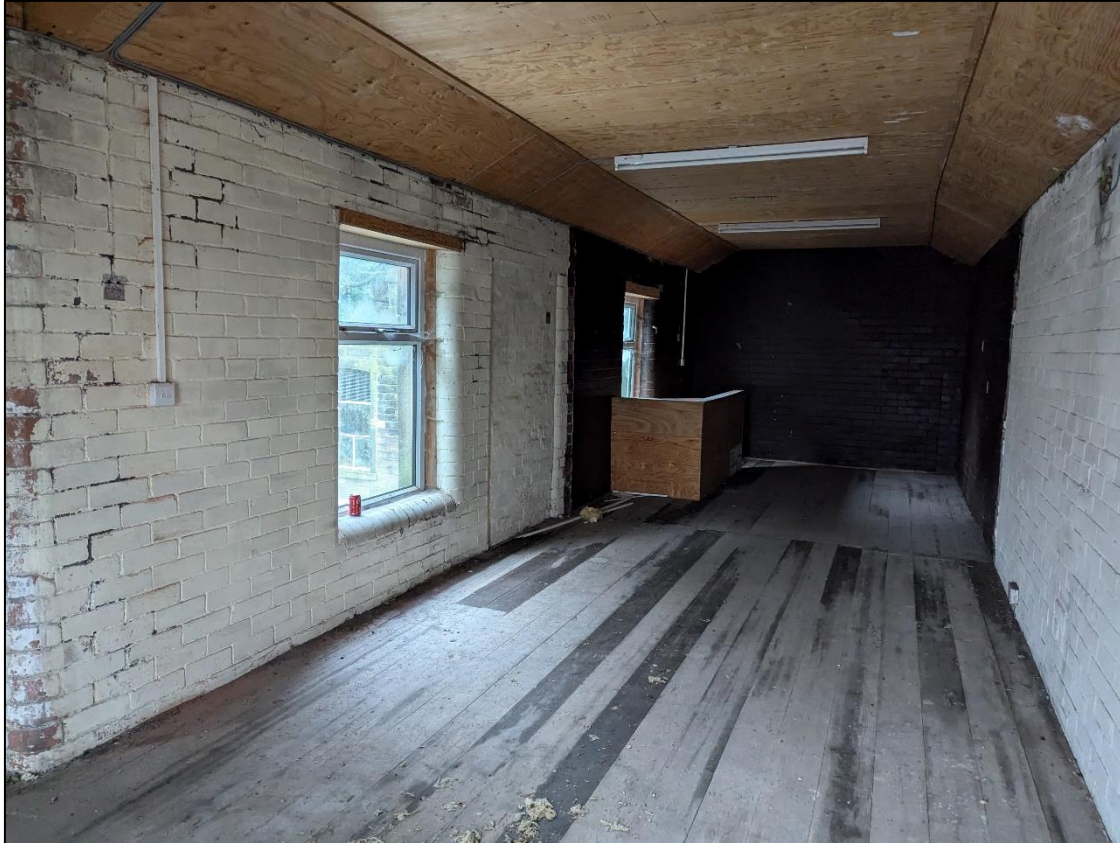
Plate 52: First floor looking north
