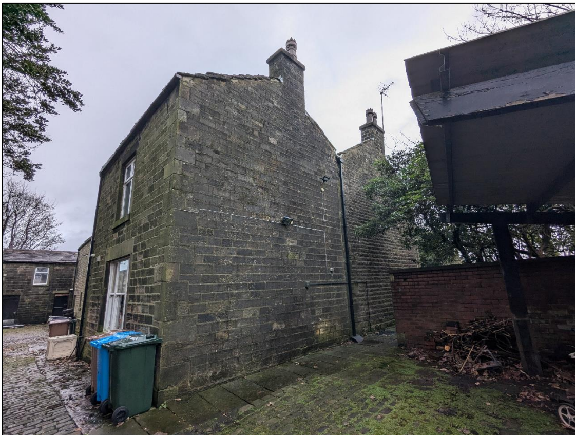
Plate 22: Double gable to west elevation of house
