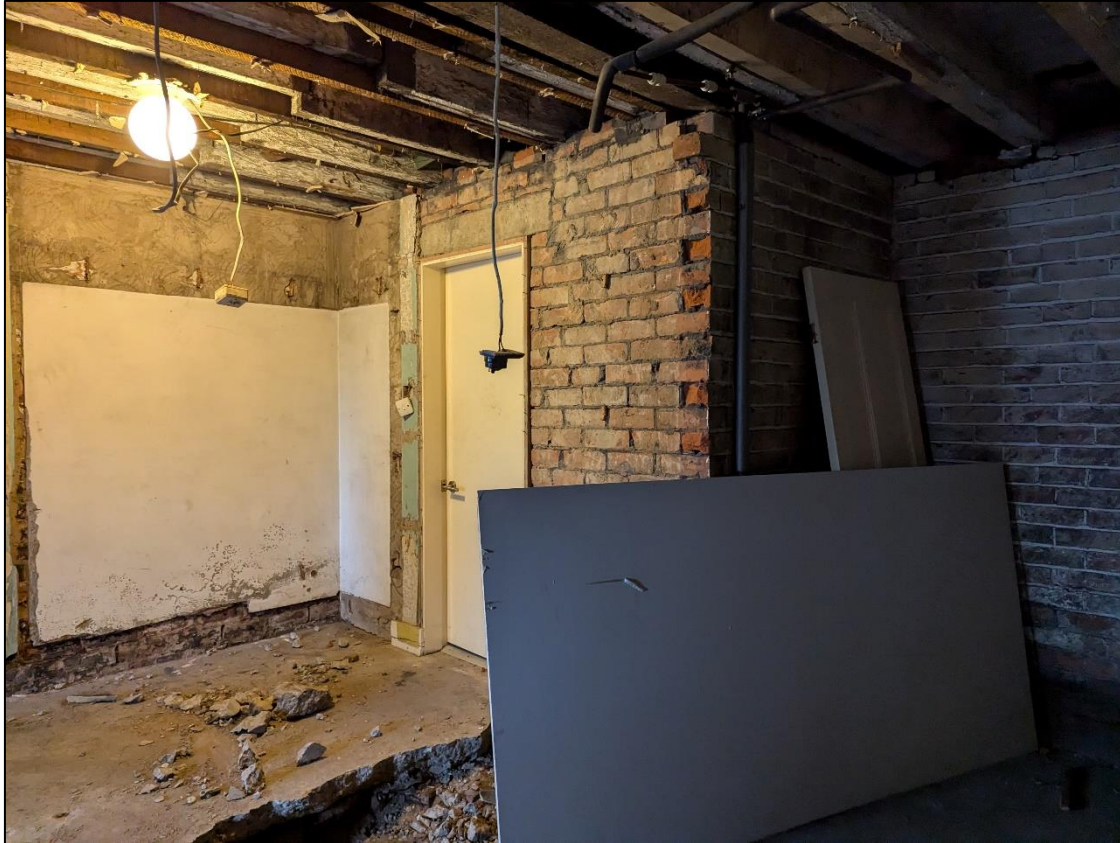
Plate 36: Inserted shower room to northern end
