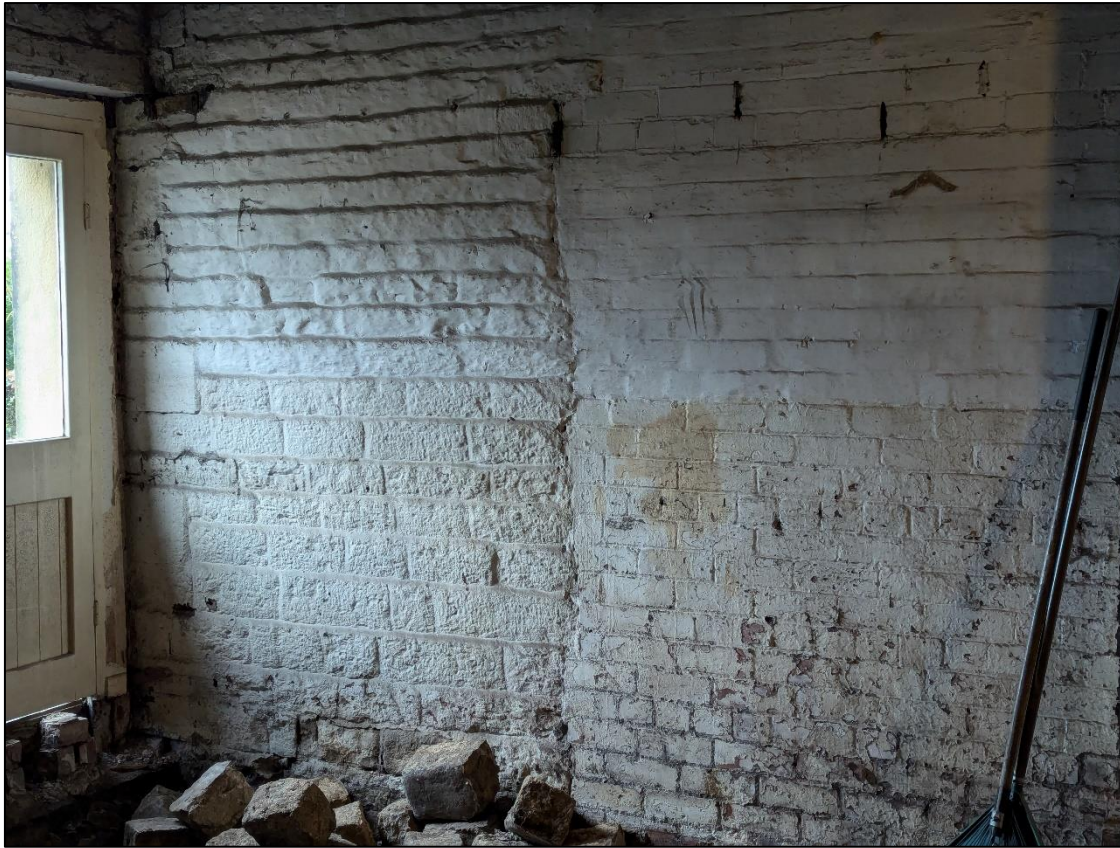
Plate 35: Detail of stonework with brick to the right
