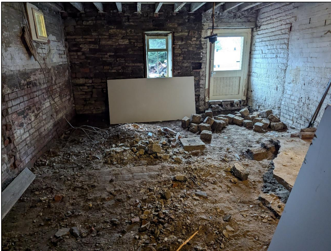
Plate 32: Ground floor of eastern bay of barn
