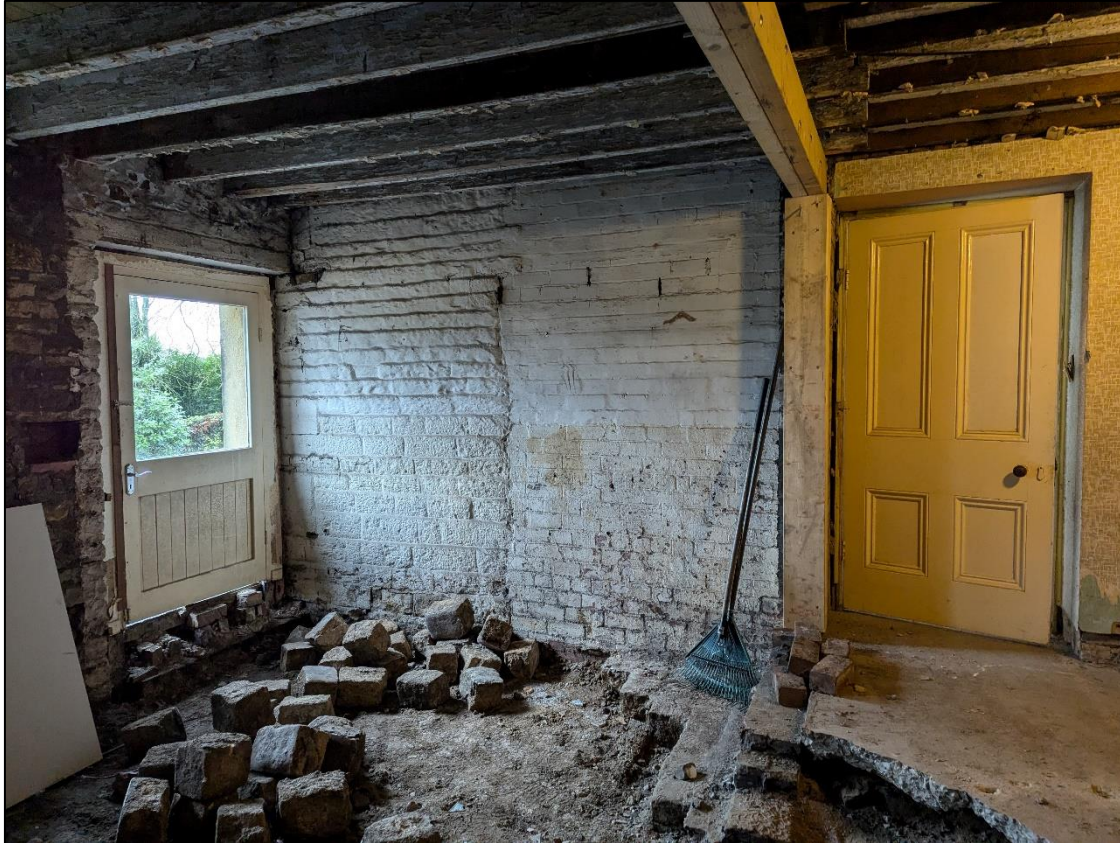
Plate 34: Eastern wall showing rough joint to stonework and inserted doorway to house
