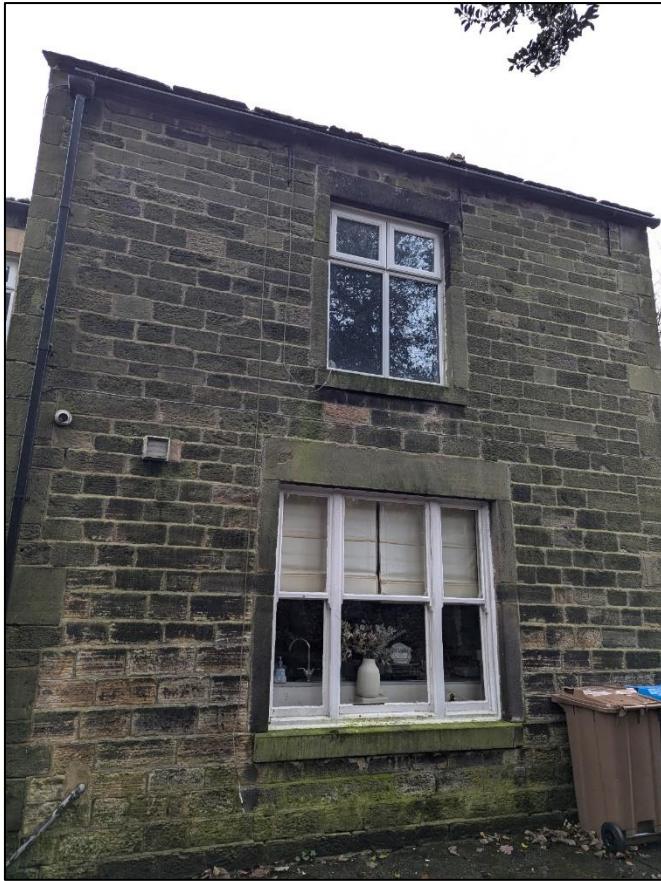
Plate 21: North elevation of projecting house extension
