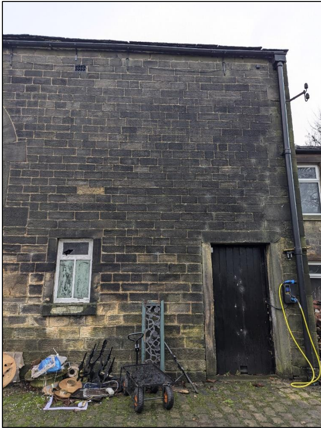
Plate 11: East end of barn showing doorway and window
