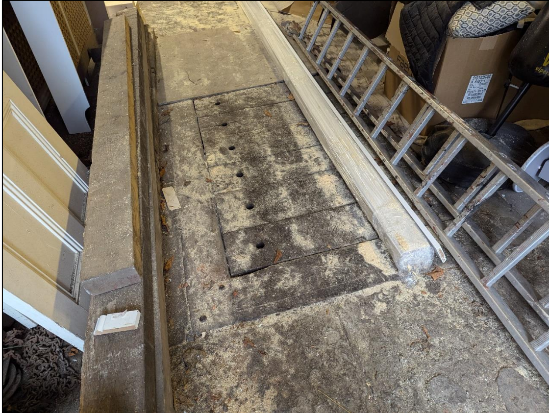
Plate 40: Inserted inspection hatch in floor
