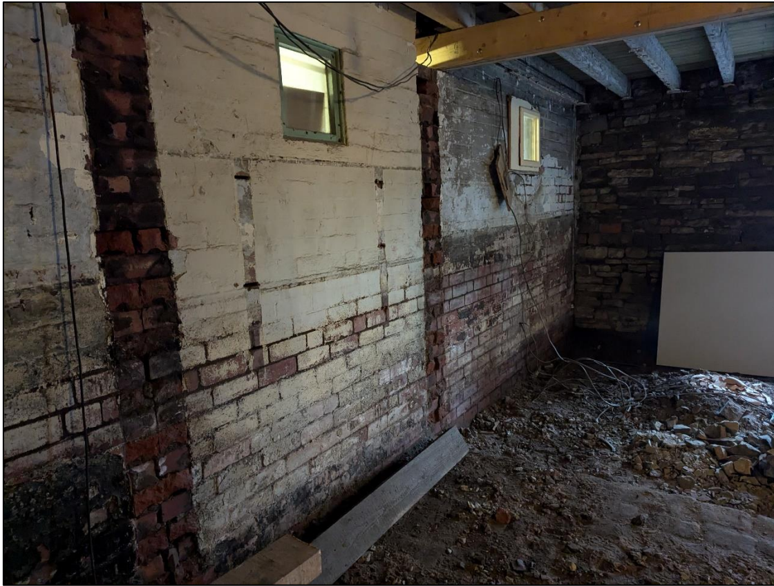
Plate 33: Inserted brick wall to central bay
