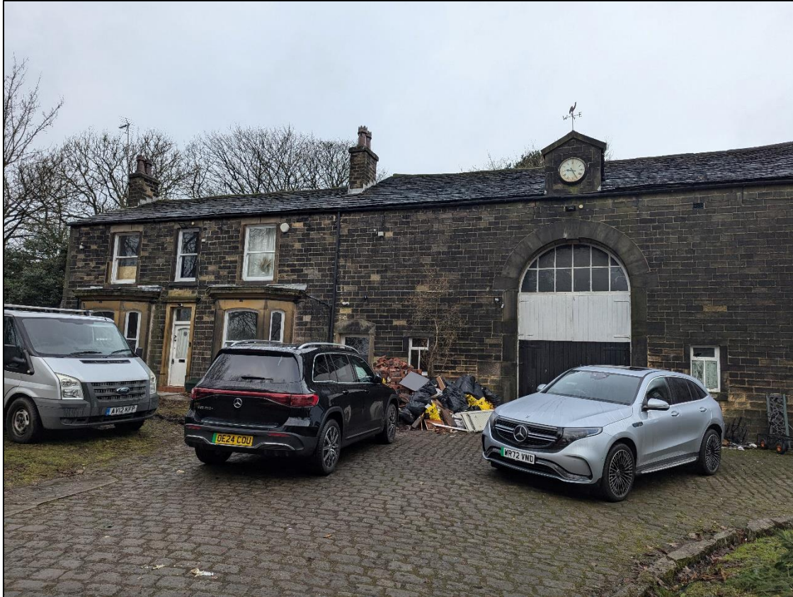
Plate 2: General shot of house and barn
