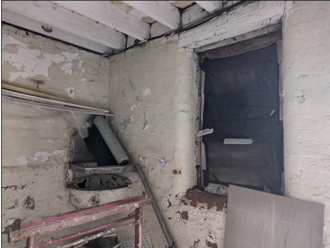
Plate 60: Bullnosed bricks to window surround
