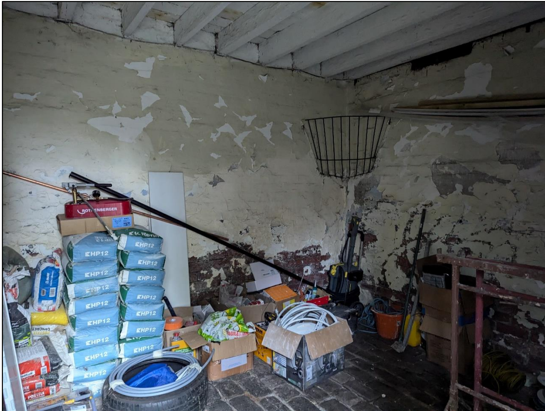
Plate 57: General shot of stable room showing metal hay trough
