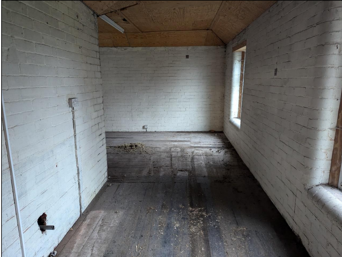
Plate 50: First floor of stable block showing brick construction
