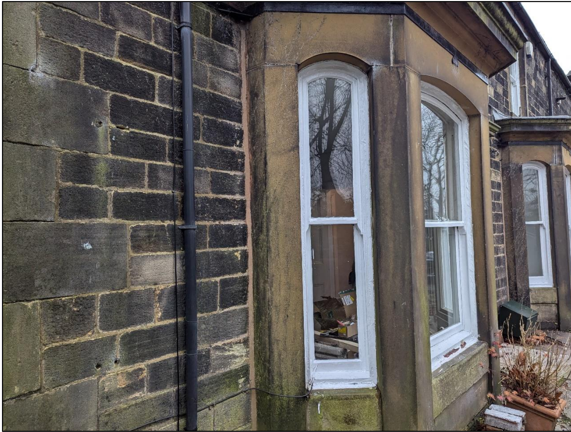
Plate 5: Bay window, stonework and quoins
