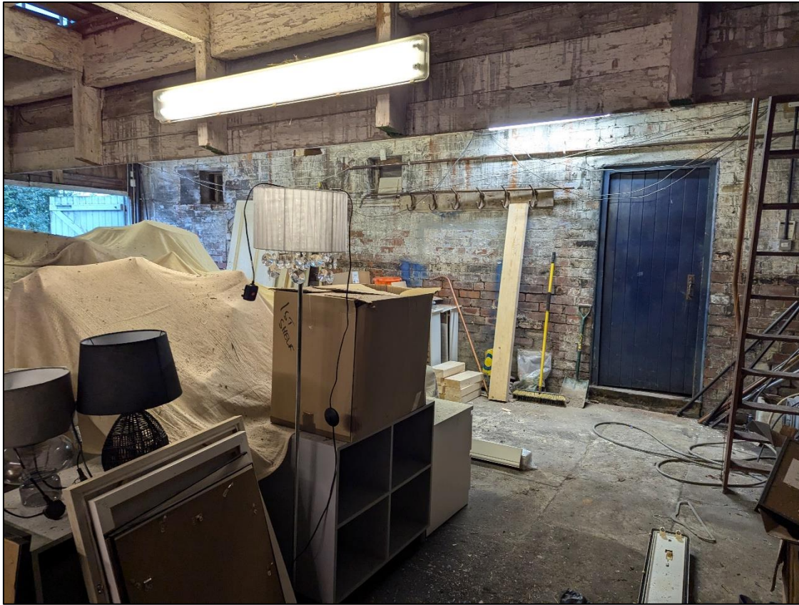
Plate 45: Inserted wall to western bay
