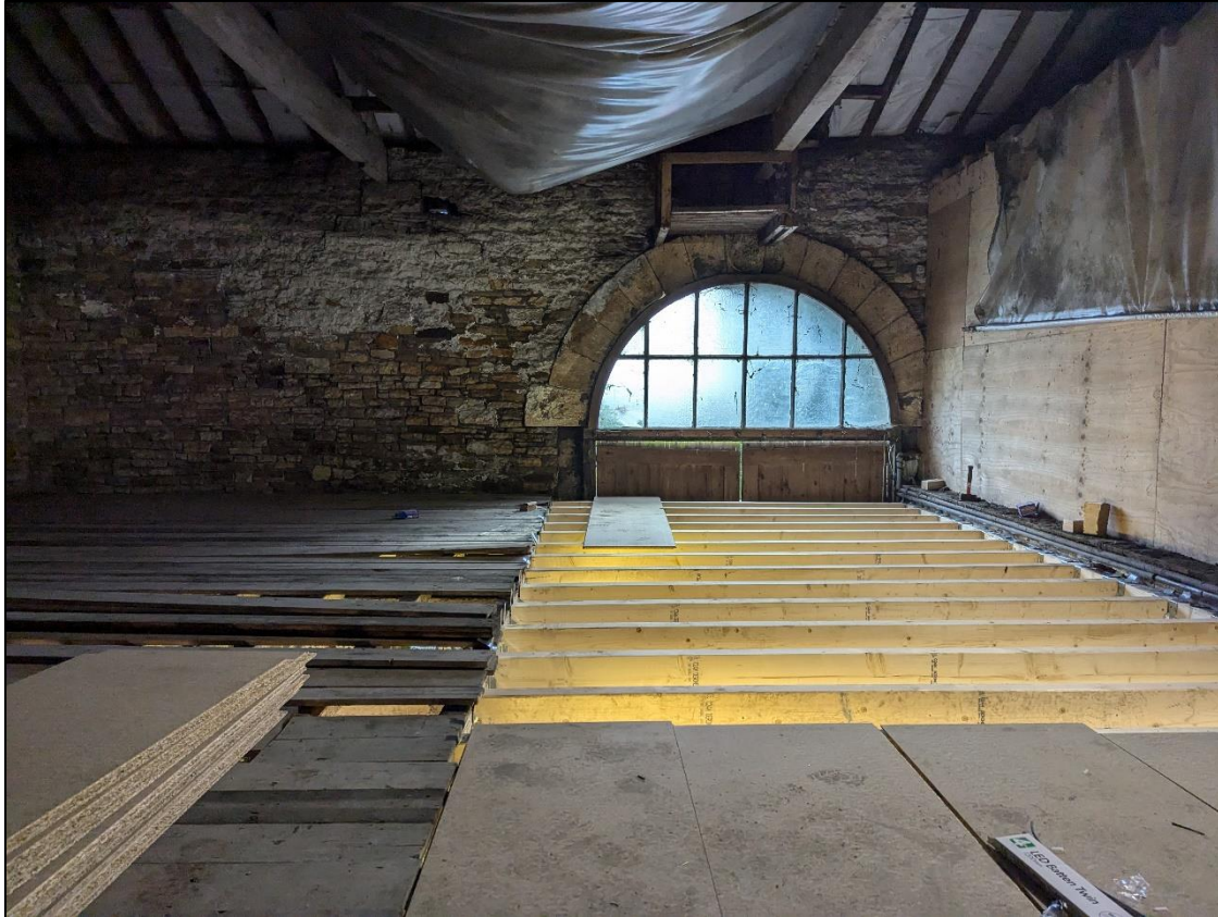
Plate 46: First floor of barn showing inserted floor cutting across doorway
