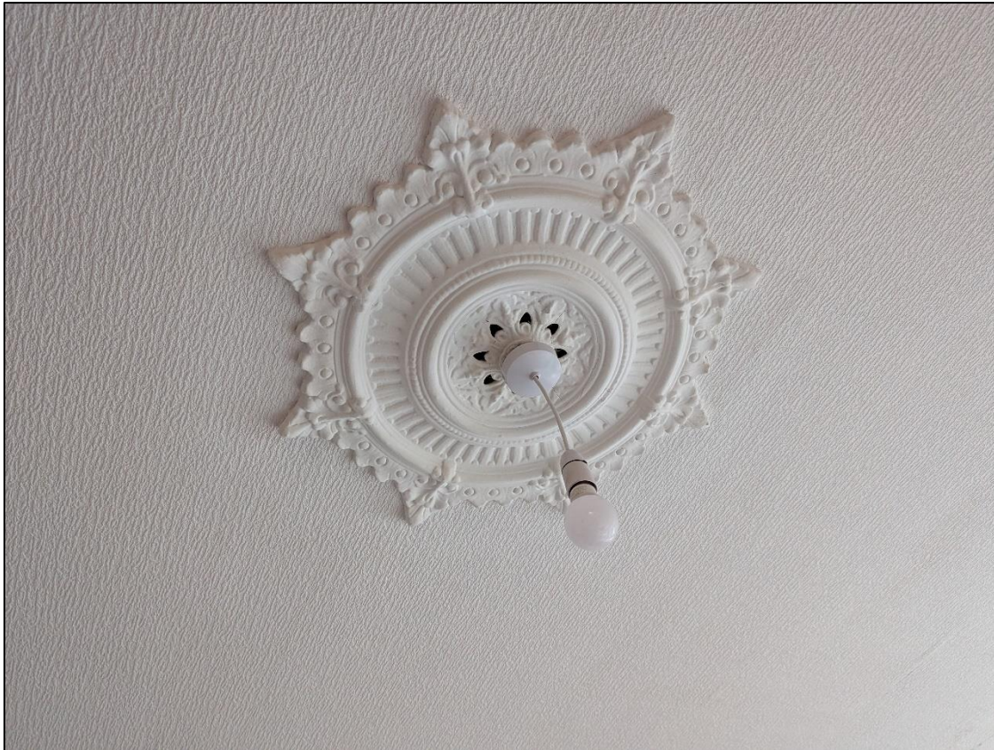
Plate 25: Ceiling rose to dining room
