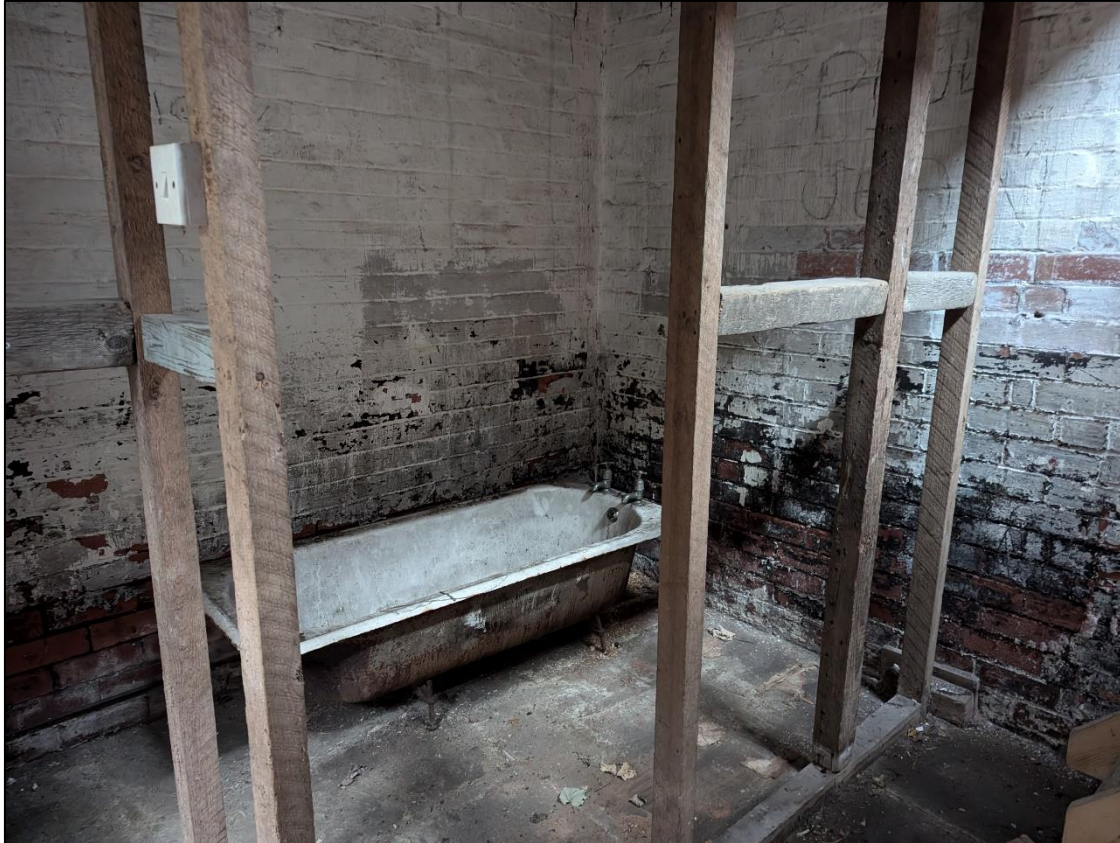
Plate 56: Inserted bathroom at northern end of ground floor
