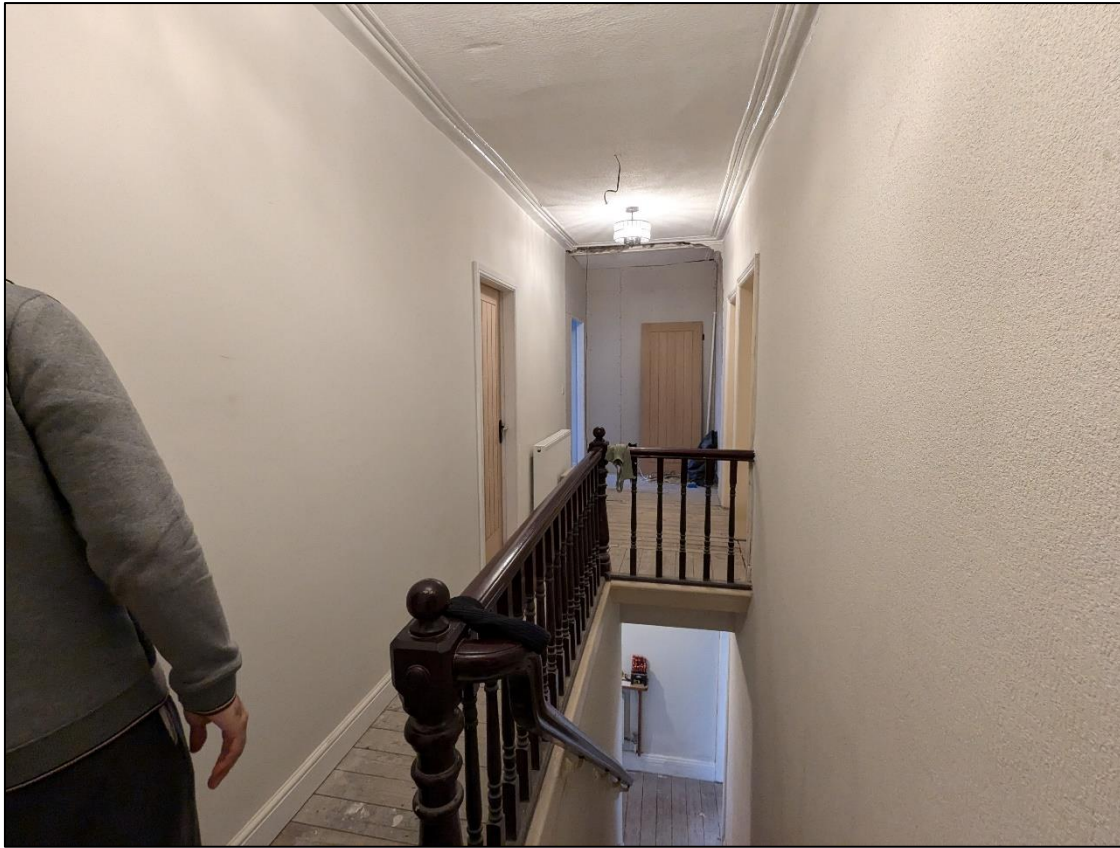
Plate 29: First floor landing
