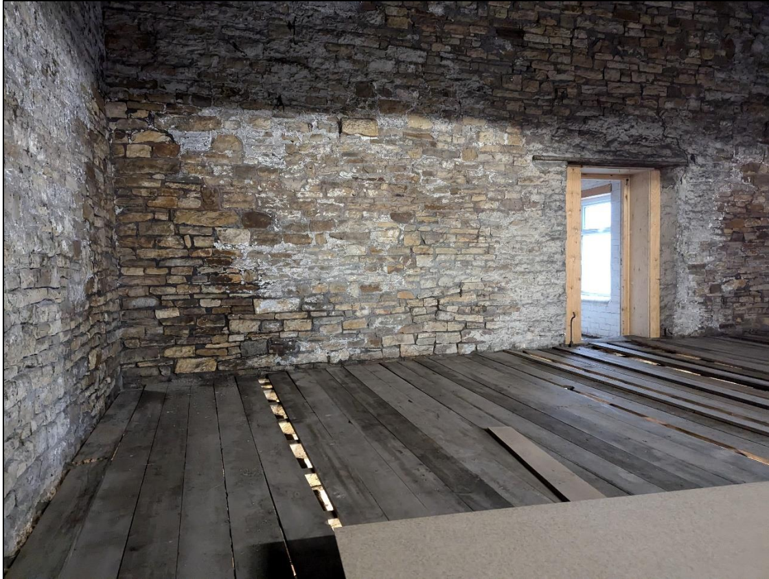
Plate 48: General shot of rough stone walling to east
