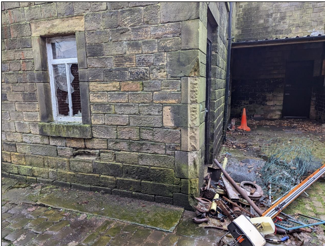
Plate 16: Detail of chamfered corner
