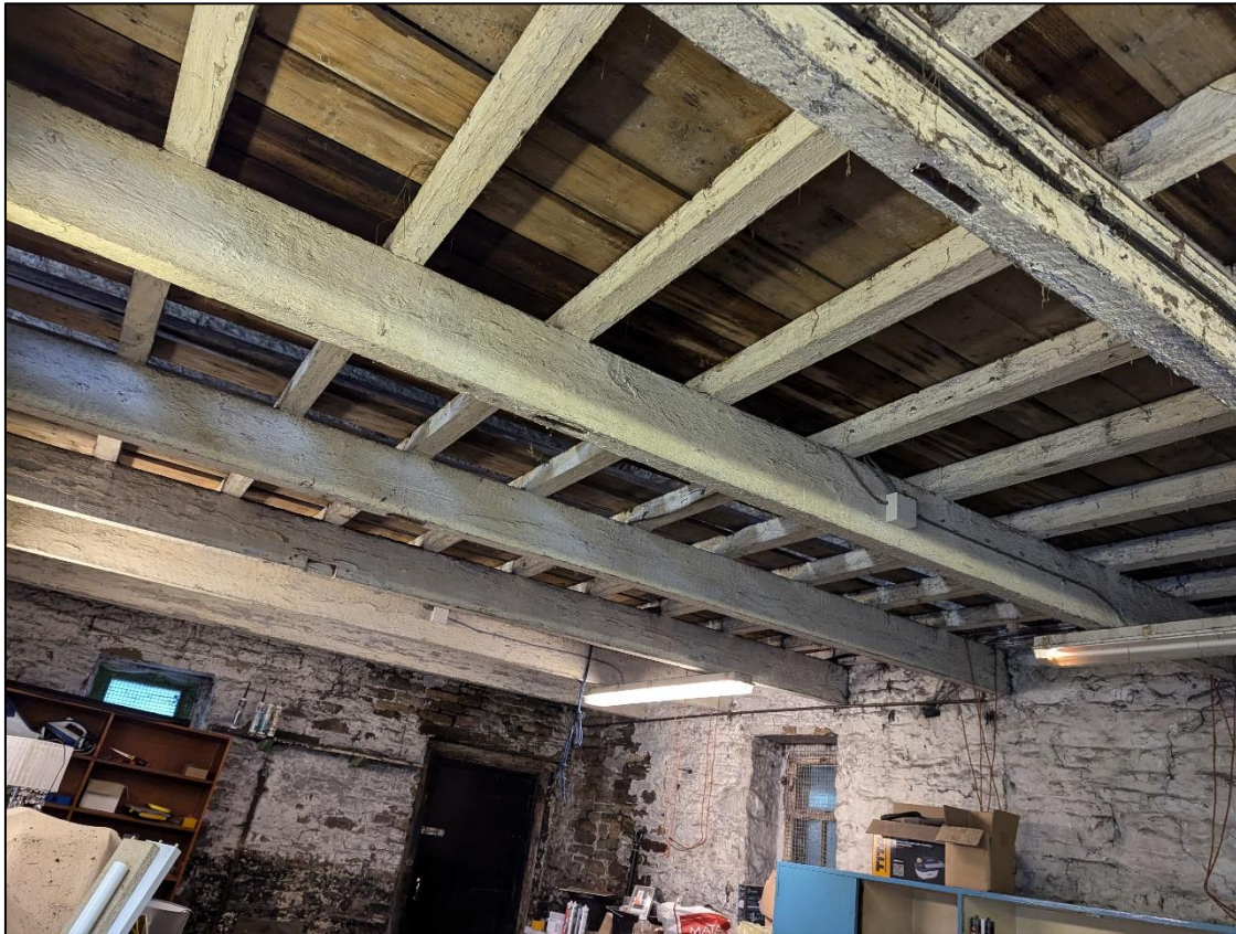
Plate 43: Timber beams with soffits to the underside
