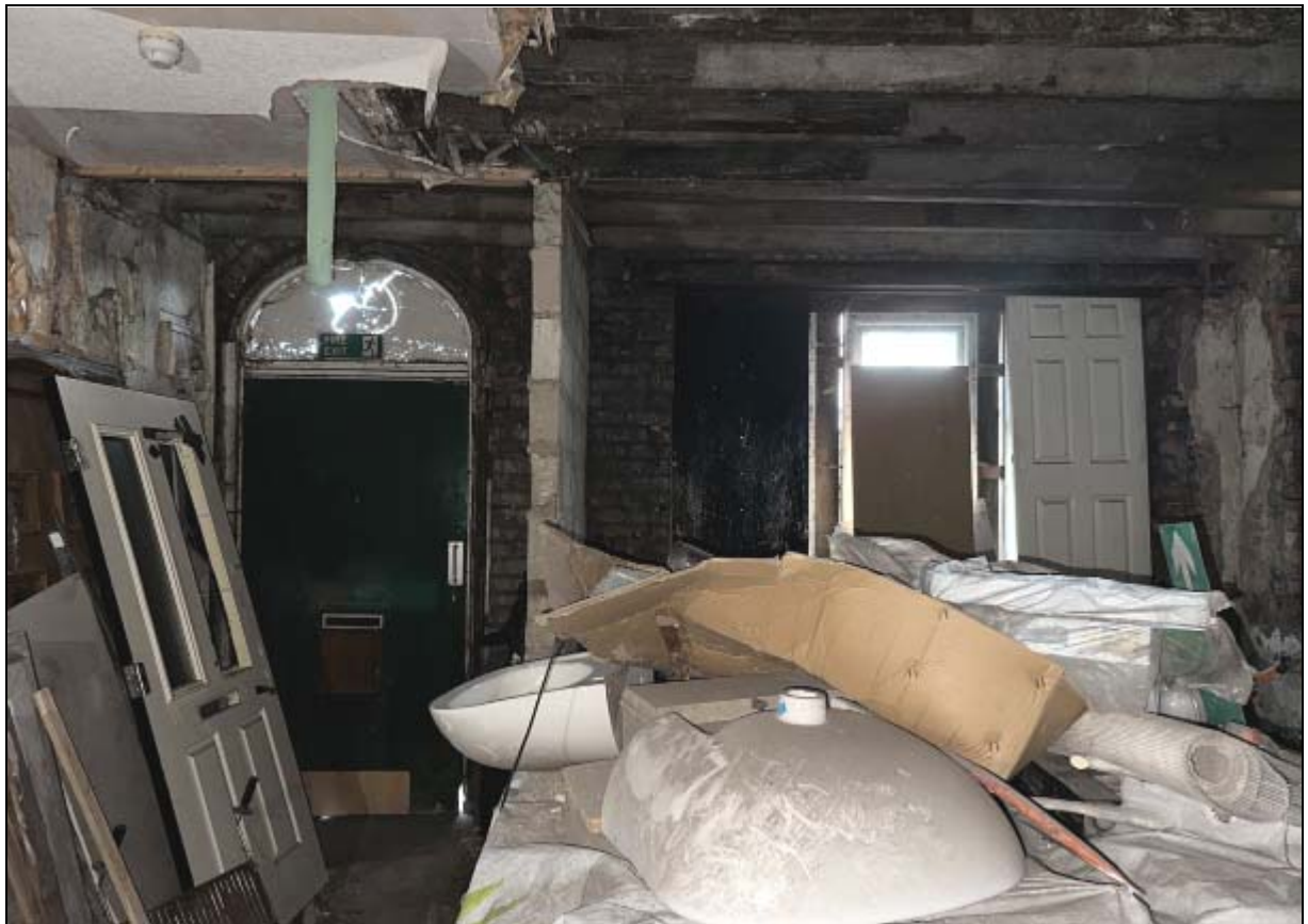
8. Interior of 190, looking to front
