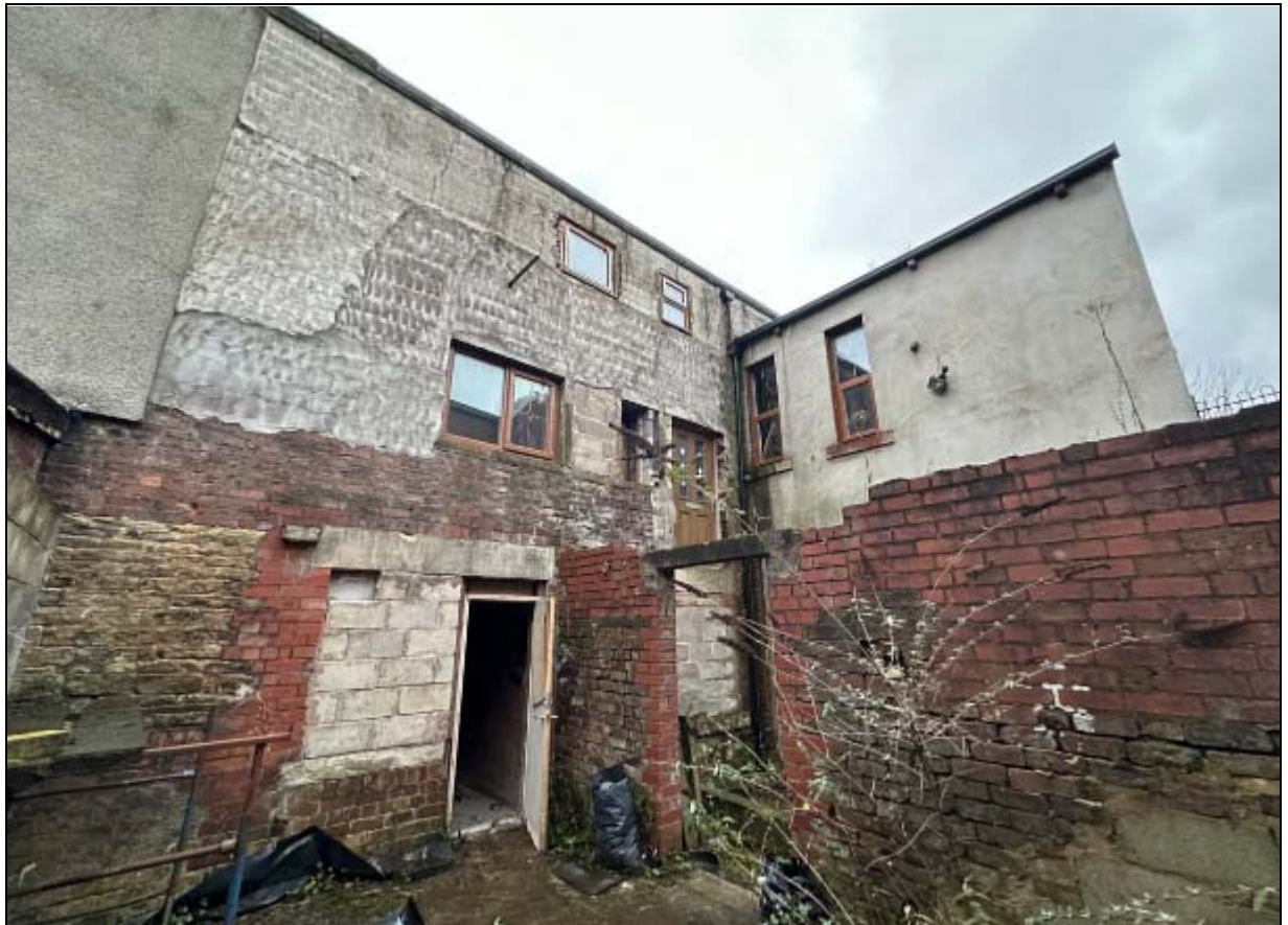
7. Rear of the properties, showing outrigger behind 190
