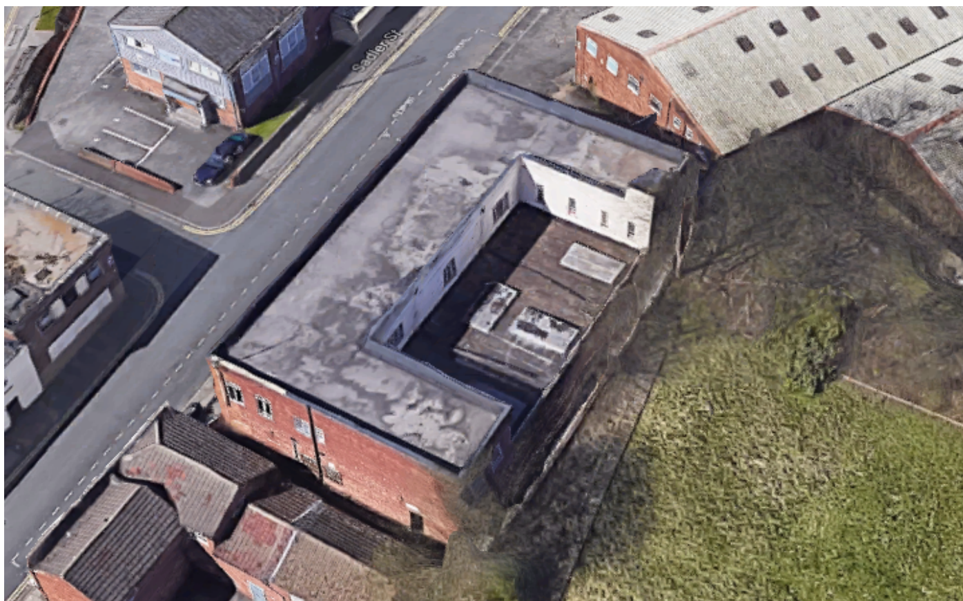
Figure 2: Existing aerial view (Rear)
