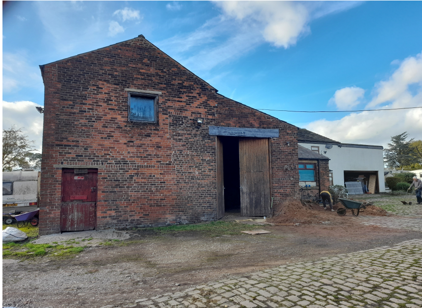
Adjoining barn on east elevation
