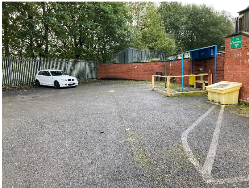
PLATE 1 SHOWING AREA OF HARDSTANDING
