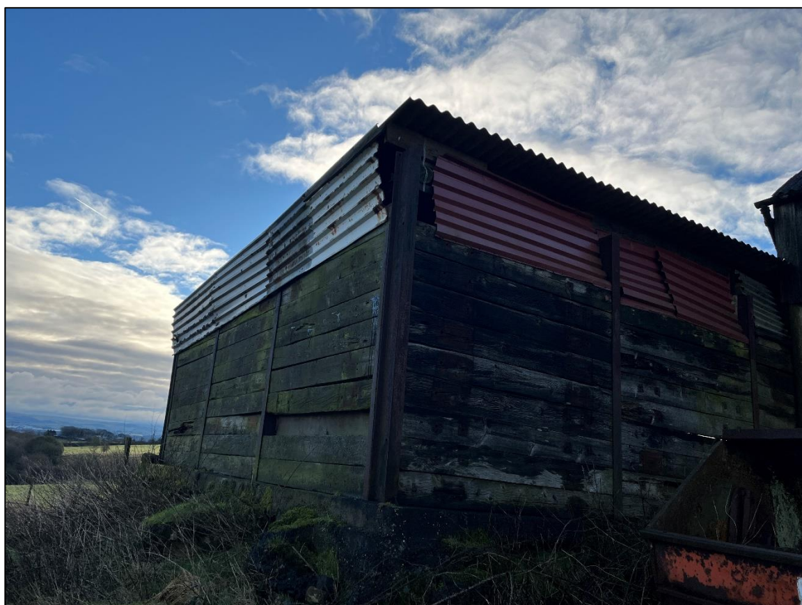
Plate 6 – Rear of eastern lean-to section of B1
