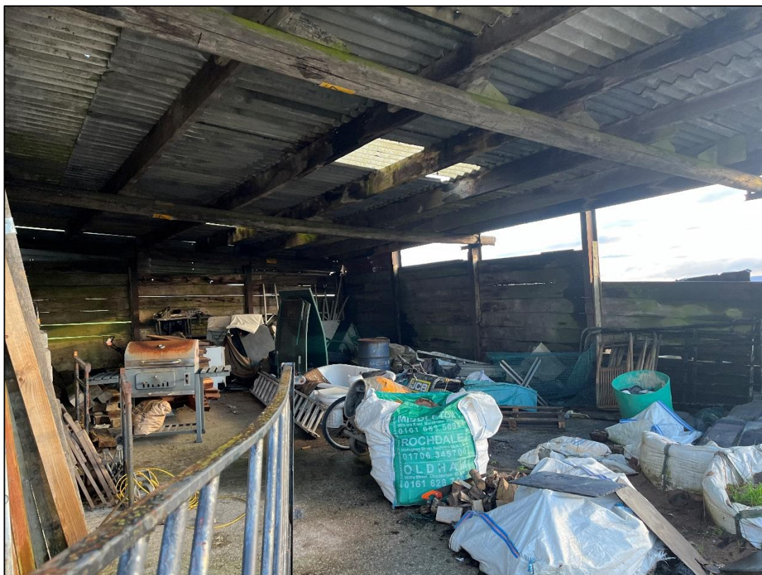
Plate 2 – Interior of the lean-to section of B1
