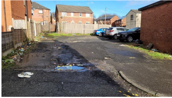
Block C – Un-made Land from the South
