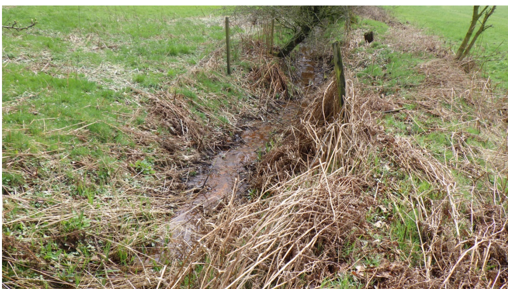
Photo 12 – Opening of water course from culvert
