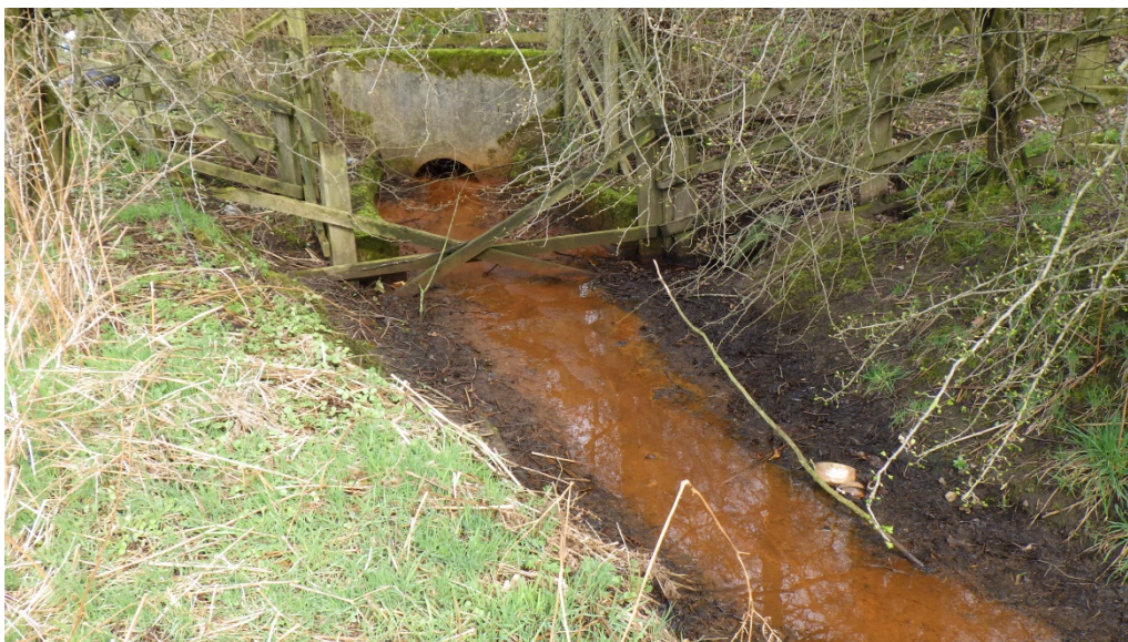
Photo 11 – Culvert located along the northern boundary
