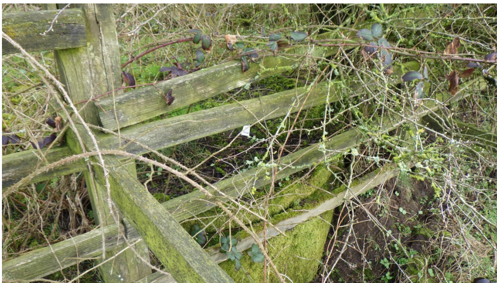
Photo 13 – Manhole located adjacent to northern boundary
