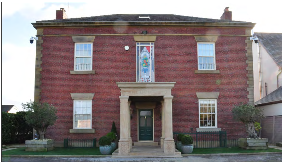
Photo 2: Dane House: rear elevation
