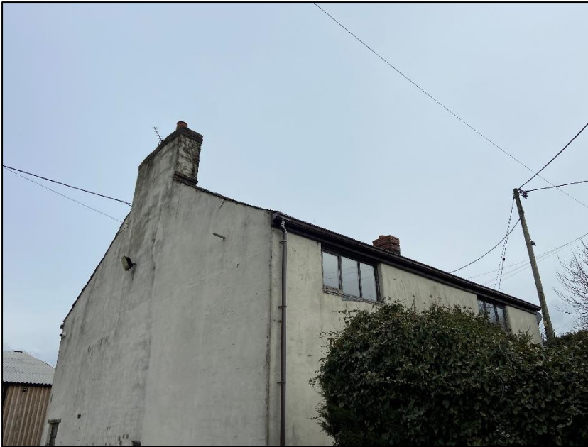
Photograph 6 showing the south-eastern and south-western elevations
