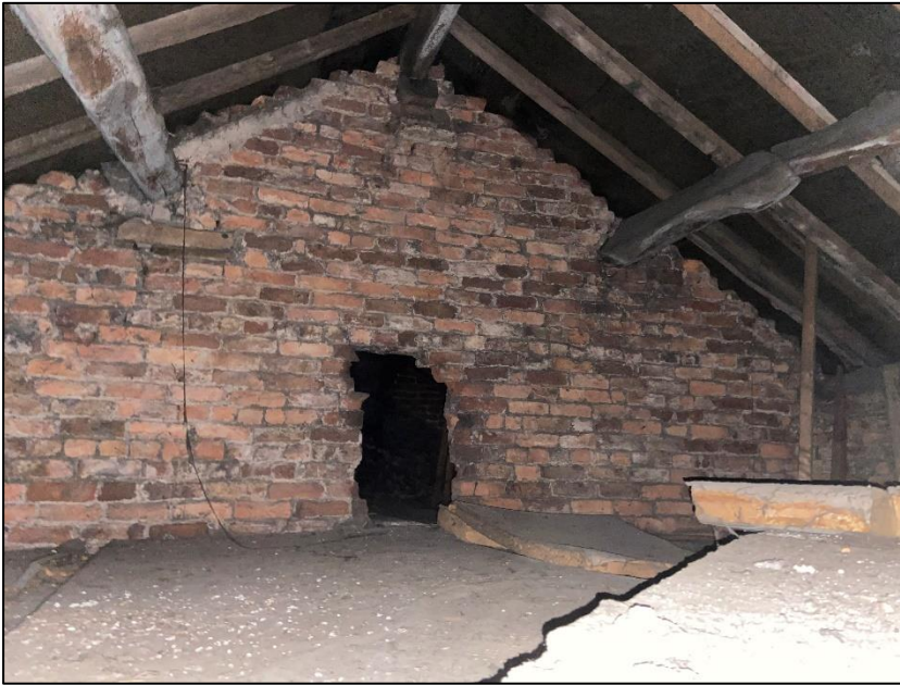
Photograph 11 showing the roof void of the property
