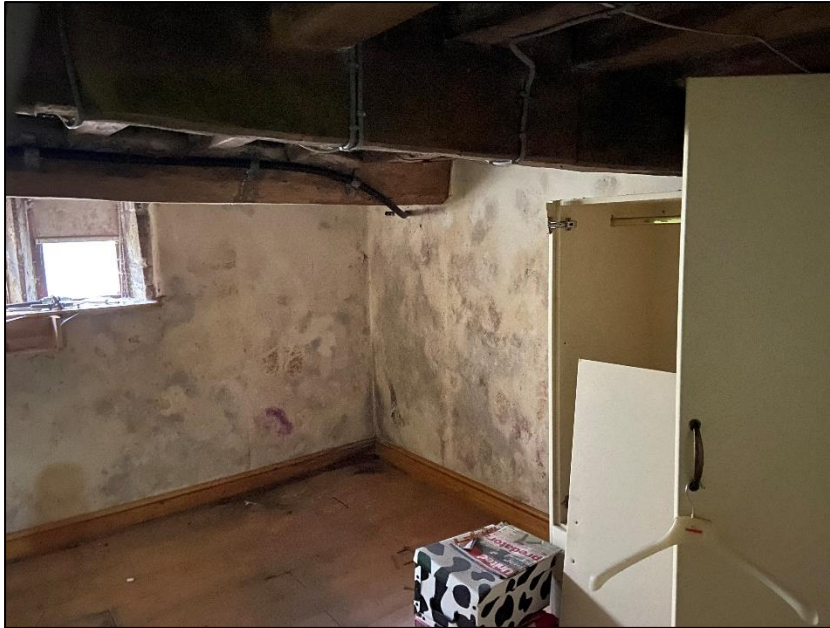
Photograph 13 showing the basement of the property
