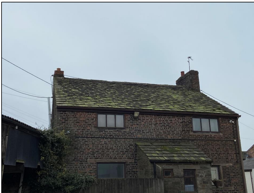
Photograph 5 showing the north-western elevation of the building
