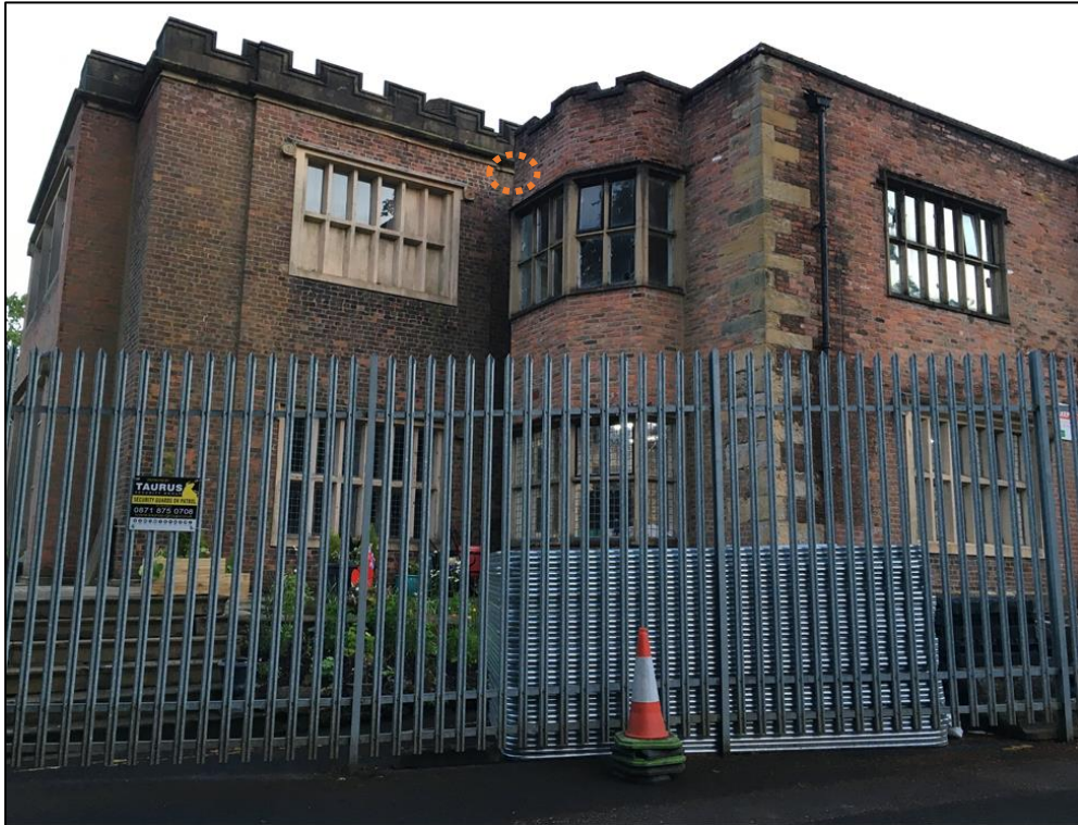
Figure 5.1 - Dusk Survey 1 & Dusk Survey 2 - Visual Aid - Emergence locations on the northern elevation; where a single Common Pipistrelle emerged from below the coping stone of the parapet wall and a single Common Pipistrelle emerged at the join of the second storey canted bay window meets the brickwork.
