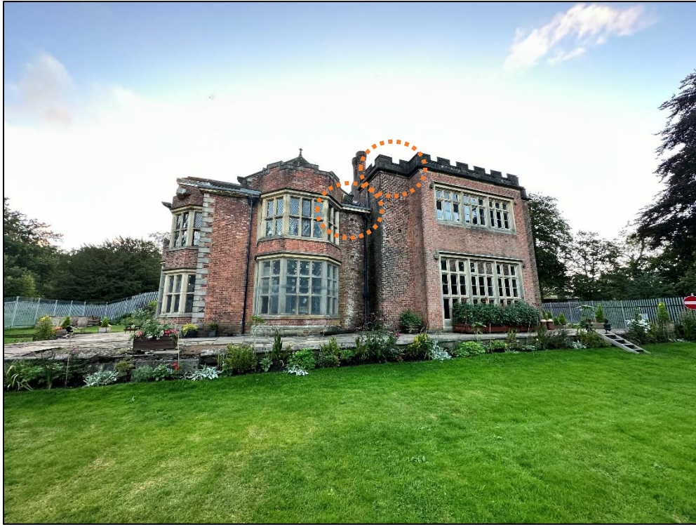
Figure 5.5 Dusk Survey 1 - Visual Aid – Emergence locations for 5 x BLE, 3 from over the parapet wall and 2 from the soffit.
