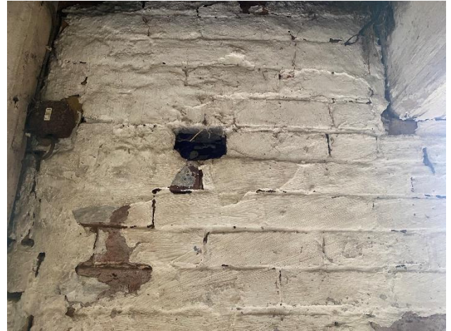
Photo 20: Missing brick within building two leading to cavity wall.
