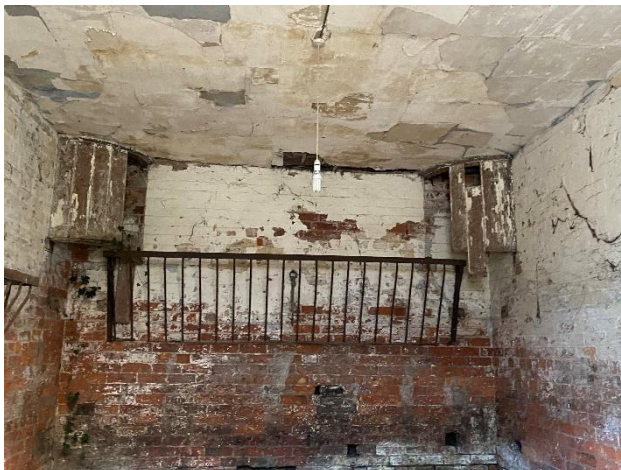
Photo 21: View of one of the stable bays located on the northern section of building two with innumerable areas of missing mortar and major hole in ceiling leading to upper floor.
