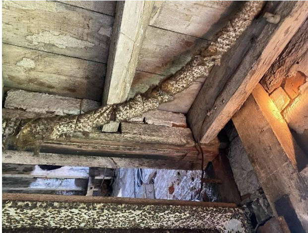
Photo 19: View internally of gaps around the beams located in the western wing of building two.
