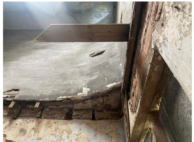
Photo 22: View of the major hole in plaster at north eastern corner of building two at high level.
