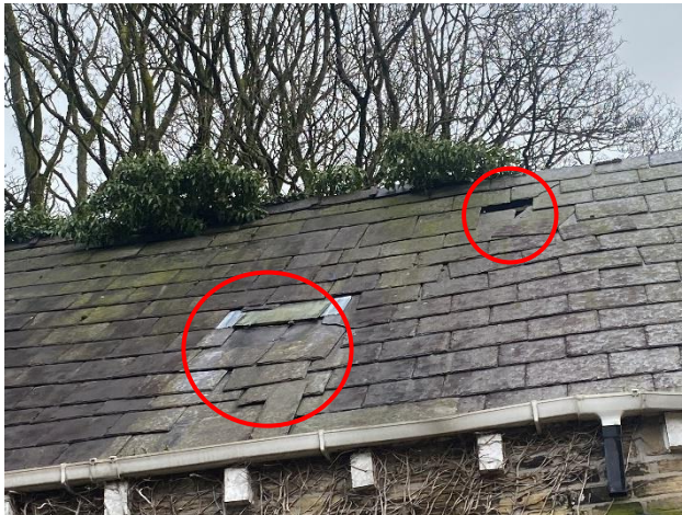
Photo 15: View of the eastern wing of building three with numerous lifted, slipped and missing roof tiles.
