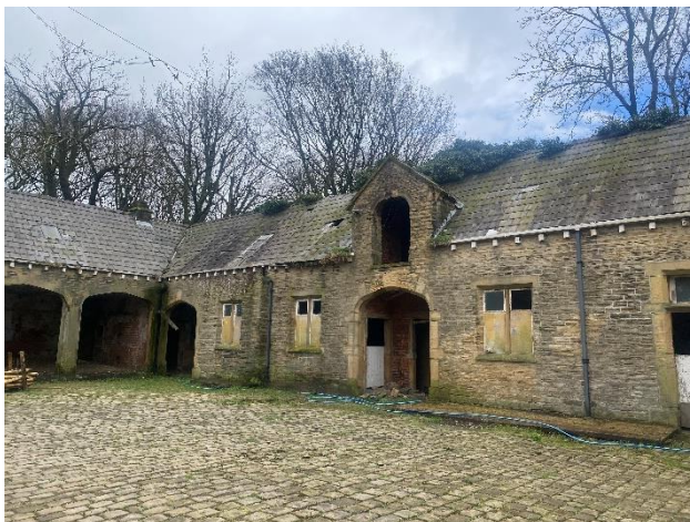
Photo 15: View of the eastern wing of building three with numerous lifted, slipped and missing roof tiles.
