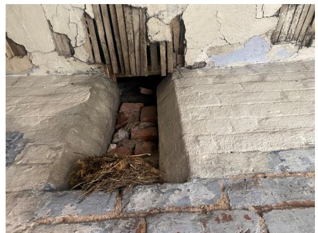
Photo 6: View of hole in the internal wall of building one leading to cavity wall, with birds nest also present.
