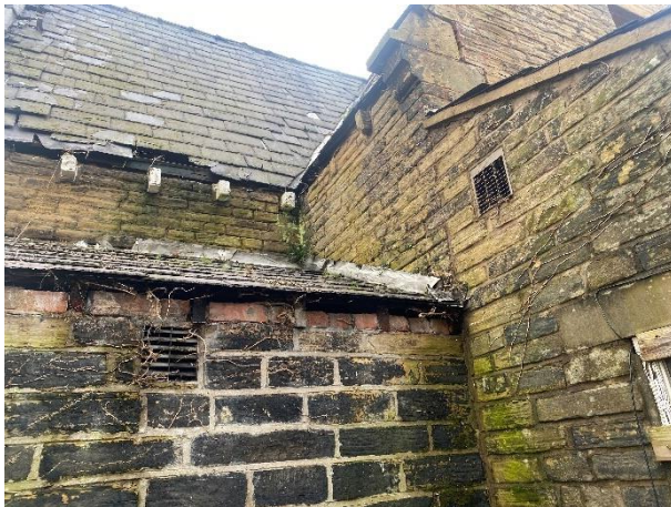
Photo 7: View of the ventilation grilles present at the south eastern corner of building two.
