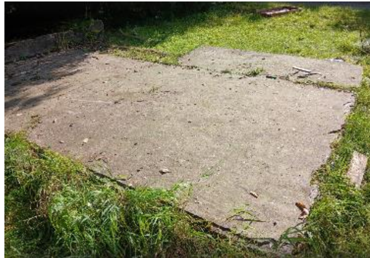
Figure 4 - View of hard standing to the centre of the site.
