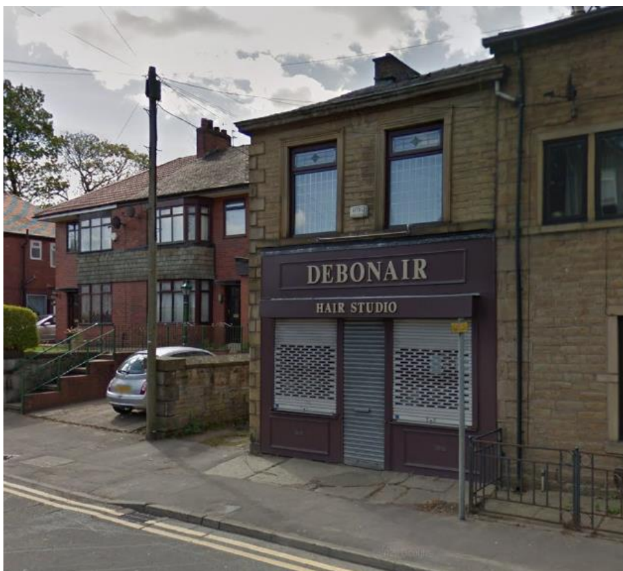
Above: Front elevation of the application site.
