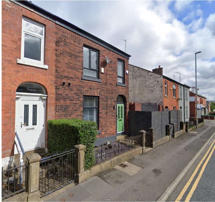
Above: Front elevation of application property.
