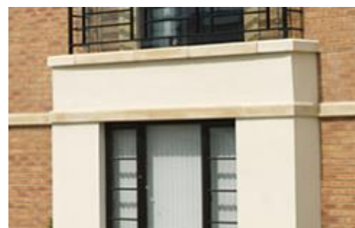
RENDER: K-REND silicone FT colour 'Champagne' with re-con stone heads and cills
