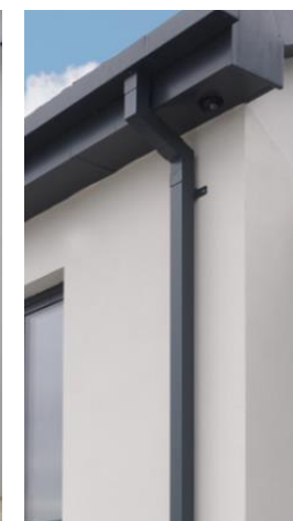
External frames, rainwater and fascias in anthracite uPVC
