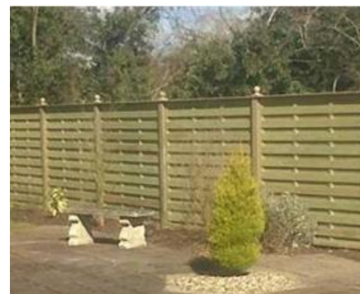
Treated timber fence panels to side & rear boundaries
