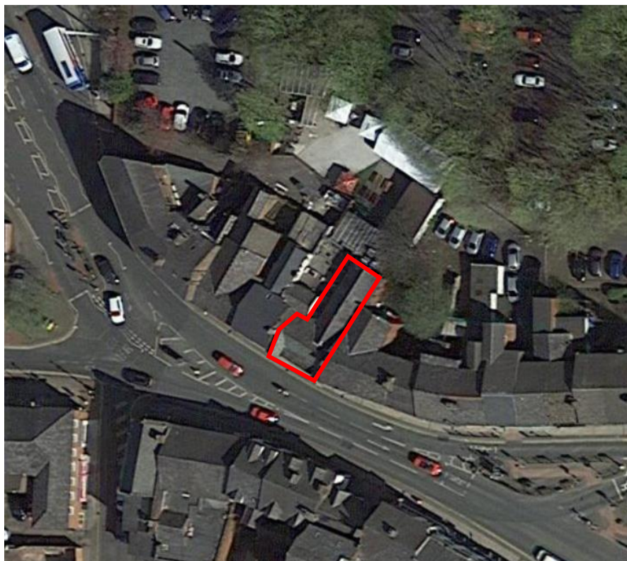
Figure 1 - An aerial image of the site in its immediate surrounding. Image source: Google
