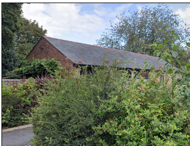
Photograph 5 Building between 56 and 64 Stakehill lane (Google Maps)
