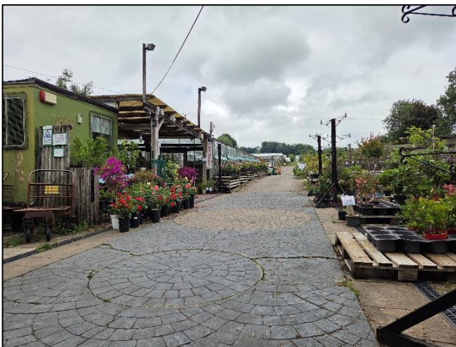
Photograph 4. Showing typical structures in the garden centre
