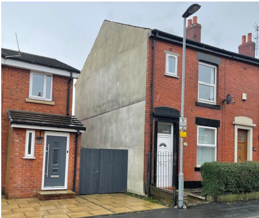
Views variously of the part-developed approved site for 07/D49154 set in between #11 Hilcrest Road and #15 / #17 / #19 Hilcrest Road
