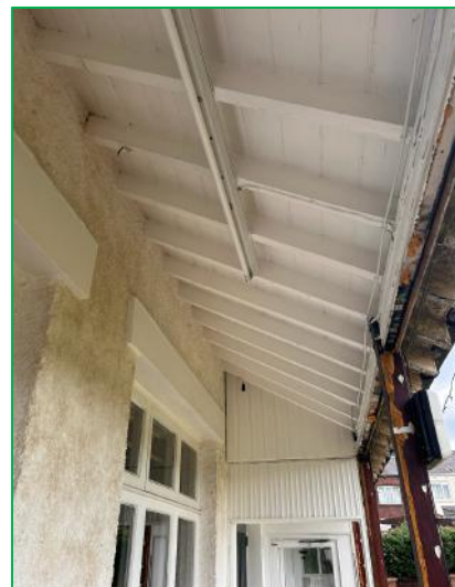
The roof overhang on the south elevation
