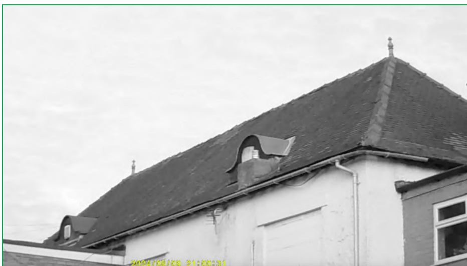
Showing the roof of the north and west elevation of the bowling club using the night vision aid.
