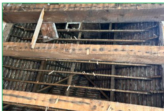
The internal roof structure of the house
