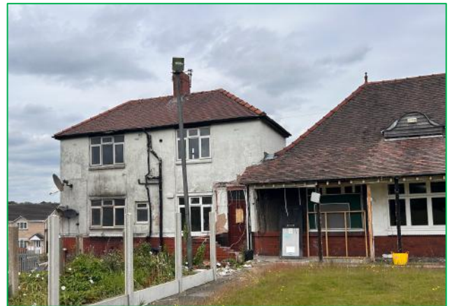
The south elevation of the house
