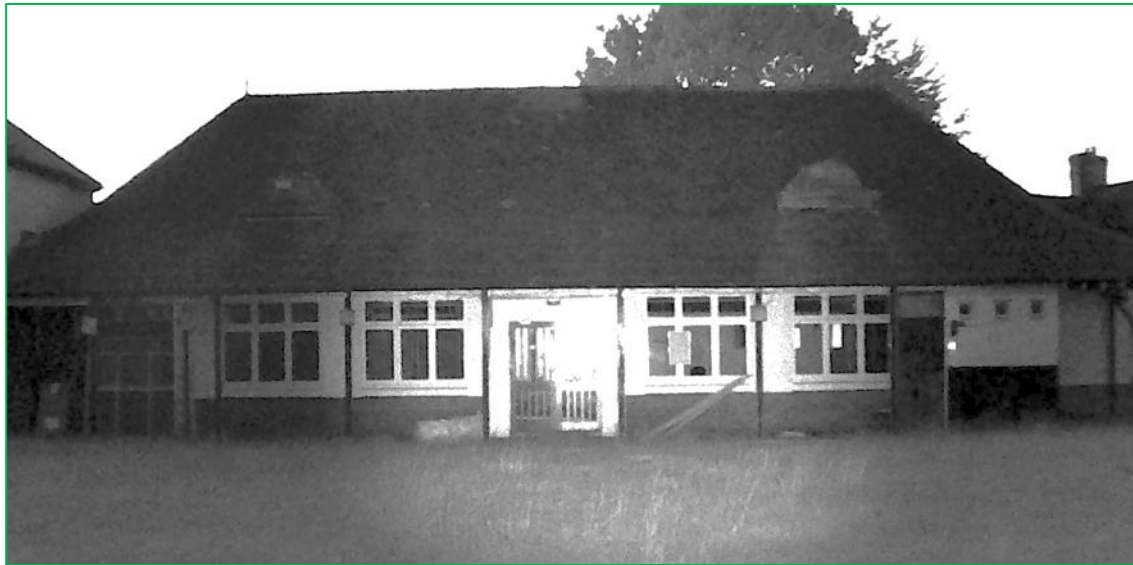
Showing the roof of the south elevation of the bowling club using the night vision aid.
