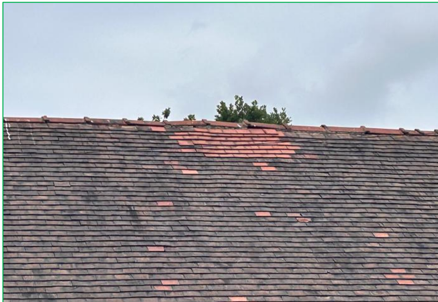
Showing raised ridge tiles on the south elevation of the building
