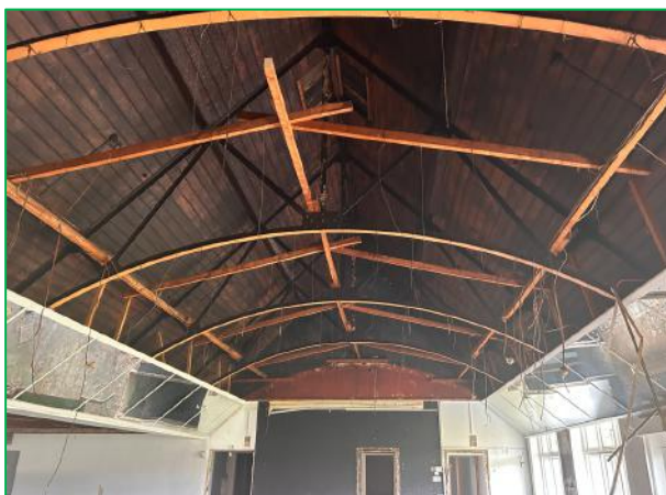
The interior roof structure of the bowling club
