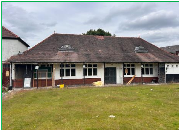
The south elevation of the bowling club
