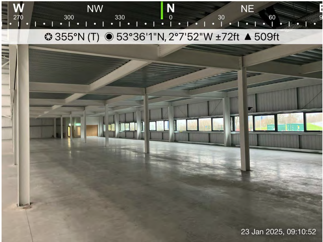
Photograph No.3: The eastern side of the warehouse has offices built above it.
