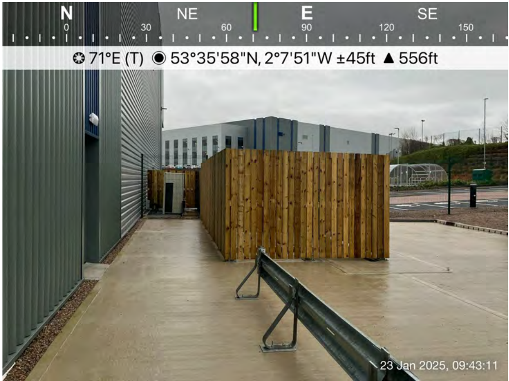
Photograph No.14: There are 3No. external storage areas bordered by wooden fencing, the 2No. in the foreground are empty.
