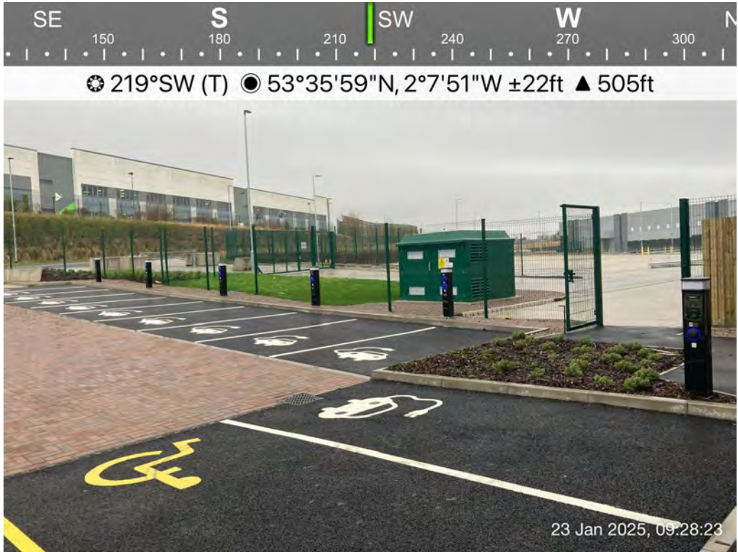
Photograph No.10: The carpark is separated from the service yard by a wire fence. There are electric vehicle (EV) charging points and an electricity substation to the southeast of the warehouse building.
