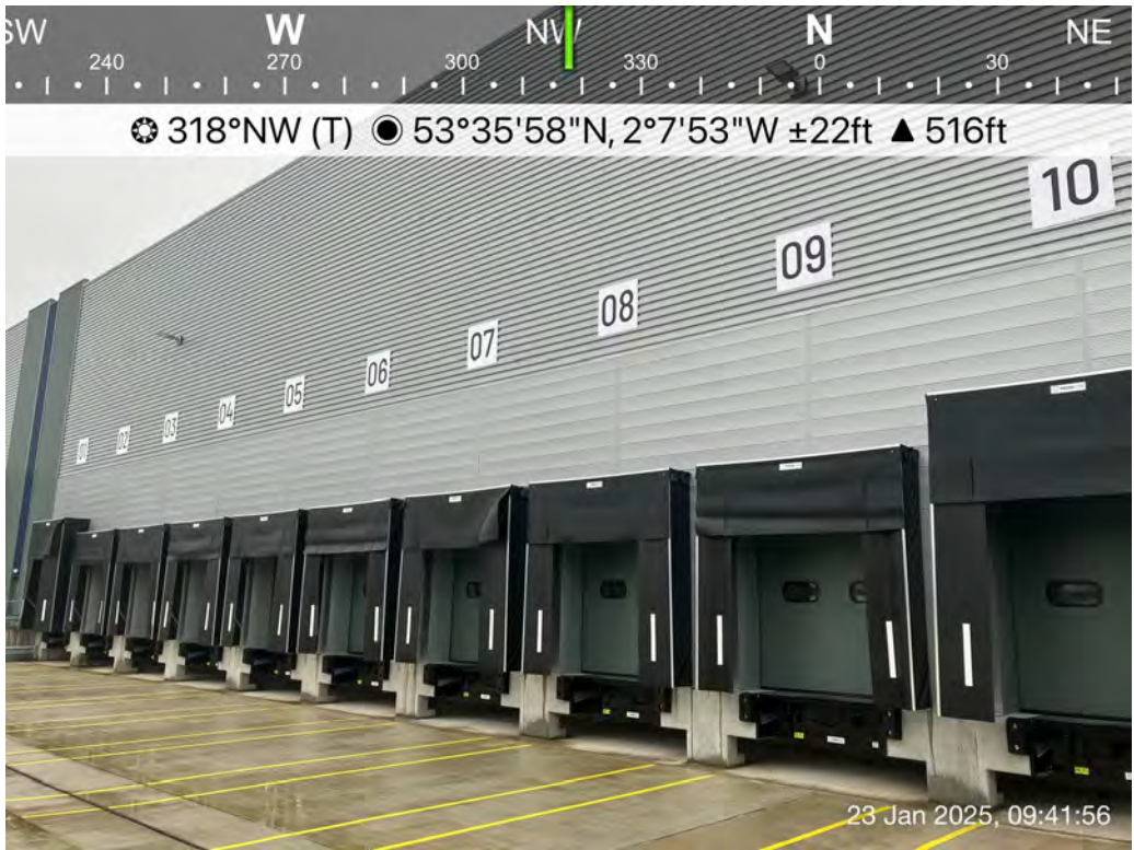
Photograph No.12: The loading bays at the front (southern side) of the building.
