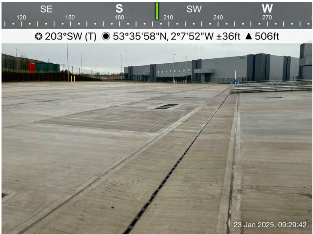
Photograph No.11: The yard dips down from the building and the road to the south. There are drainage channels through the centre and a possible interceptor in the forecourt.
