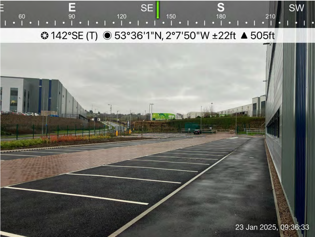
Photograph No.18: The car park to the east of the building.
