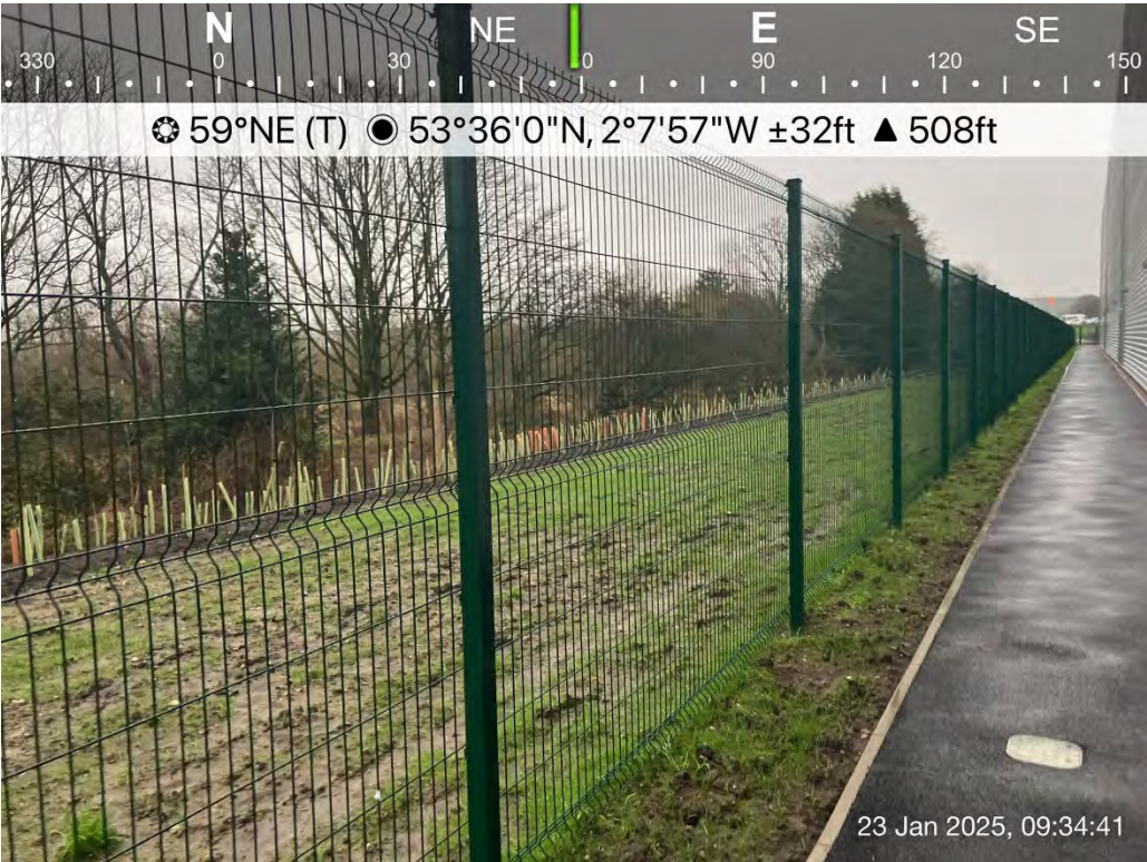
Photograph No.17: The entire site is bound by a wire fence, roughly 2m in height.
