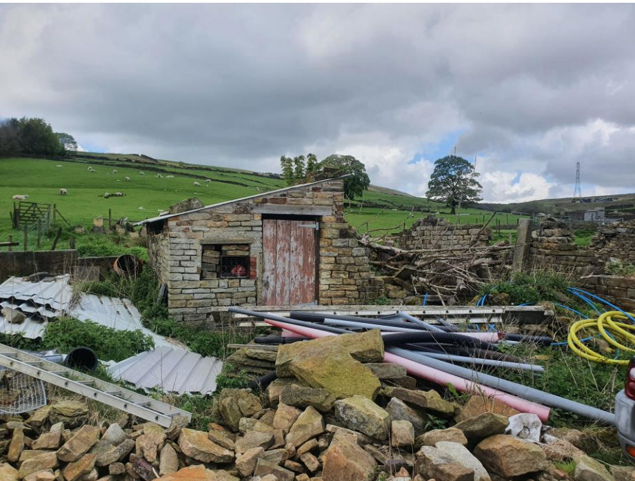
Below: Existing store, remaining barn walls & ground rubble
