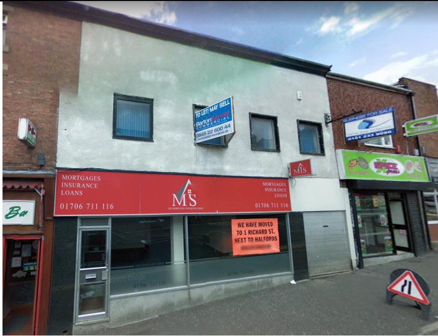
Front of application Site.
