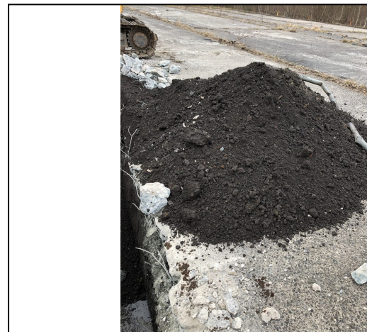
Trial Pit 110 Spoil
