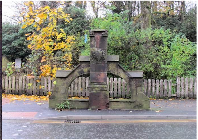
East Face of Structure
