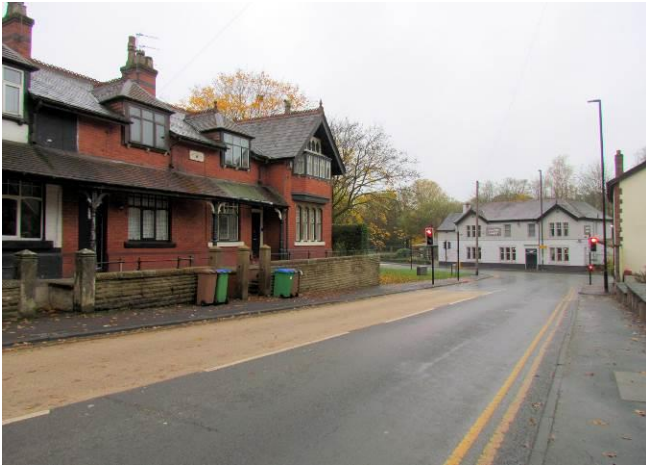
View West Along Langley Lane with Birch Villas on the Left and the White Hart in the Distance
