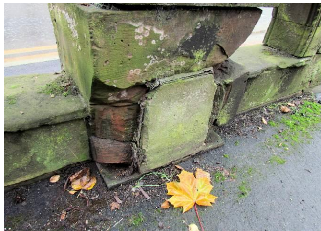
Base of Pier
