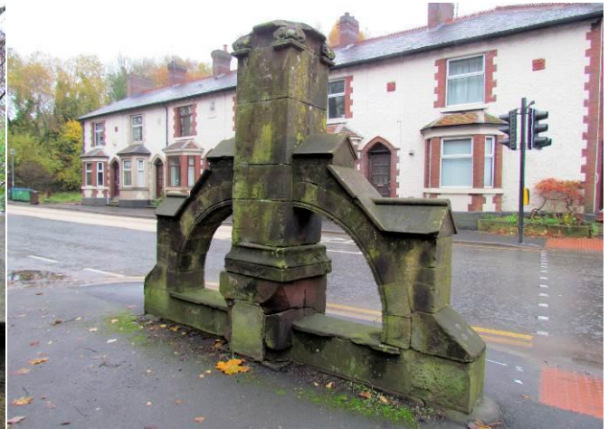
East Face of Structure
