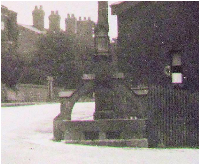
Historic Appearance of Structure, ca. 1910
