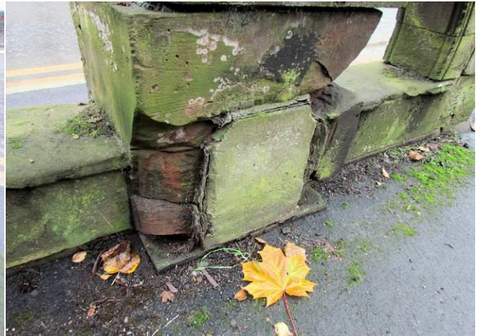
Repair in Cement Mortar
