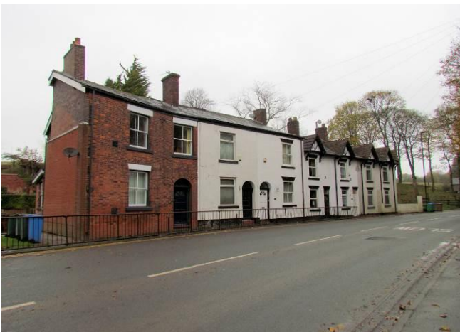
View North Along Heywood Old Road with Drywood Cottages on Right
