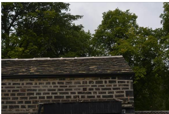
Figs. 3 & 4 Raised tiles on barn roof
