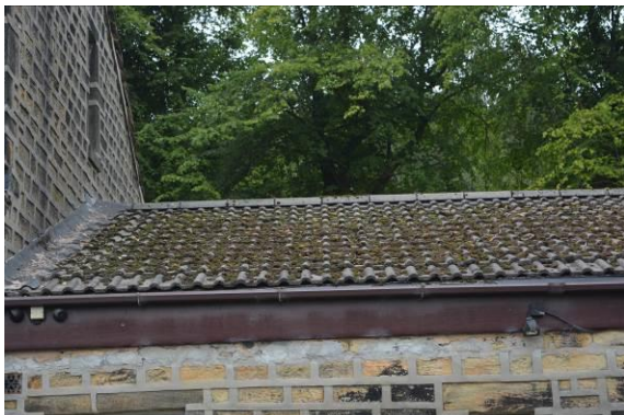
Figs. 5 & 6 Gaps beneath ridge tiles (stables)
