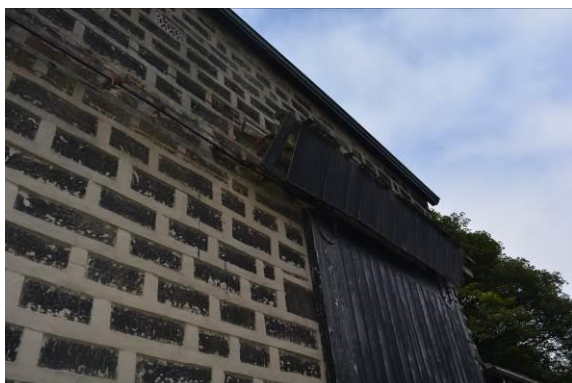
Figs. 7 & 8 Potential access points – loose door and window gaps
