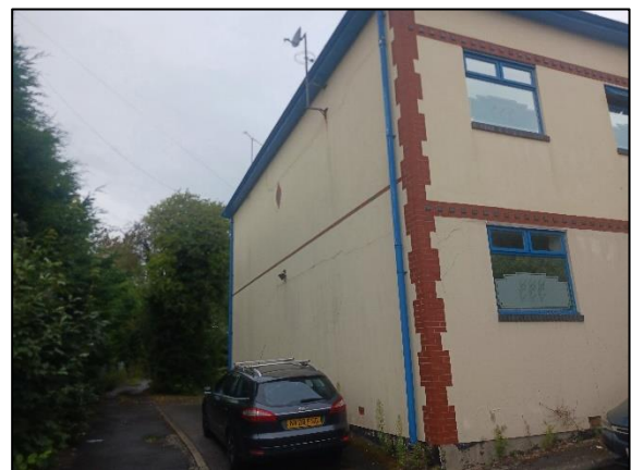
Figure 2.3: View of the south elevation of the building.
