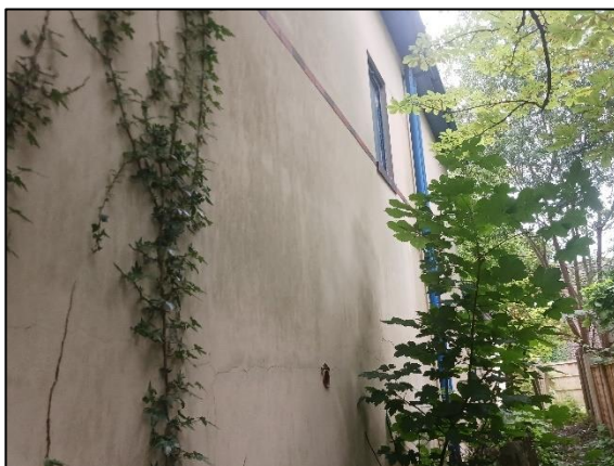
Figure 2.4: View along the north side of the building.
