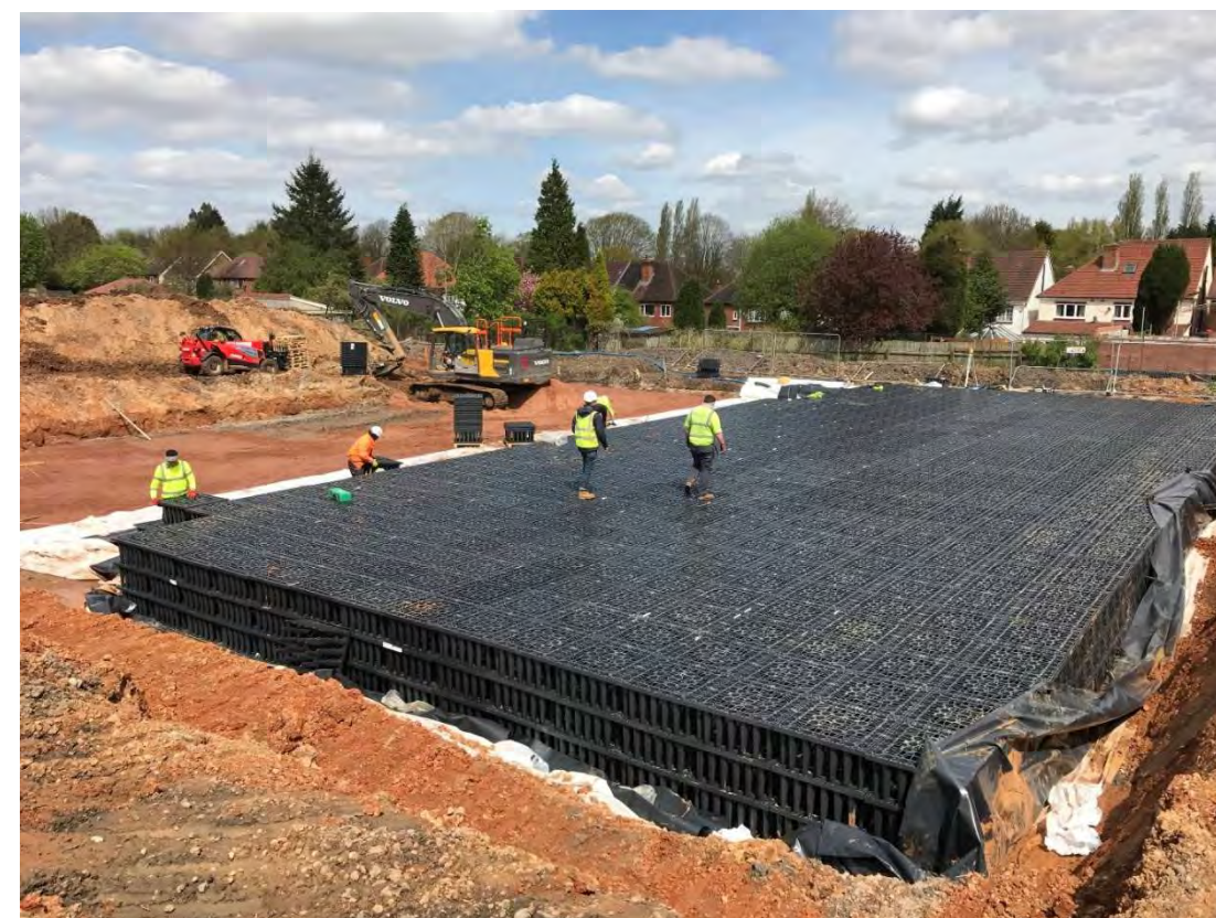
Figure 18 - Below ground attenuation
