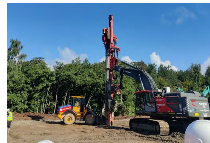
Figure 10 - Driven piling arrangement
