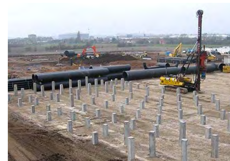
Figure 10 - Driven piling arrangement
