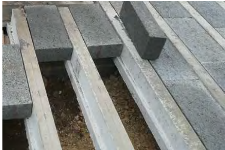
Figure 12 - Beam and block floor
