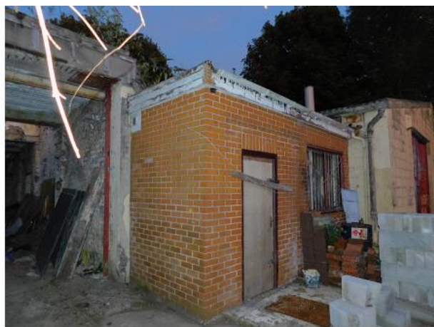
PHOTO 8 North-western Corner of Building 3
