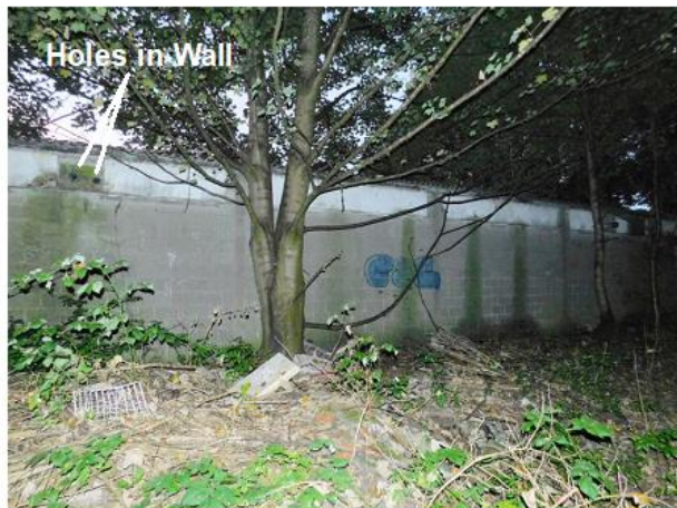
PHOTO 12 Southern Elevation of Building 4
