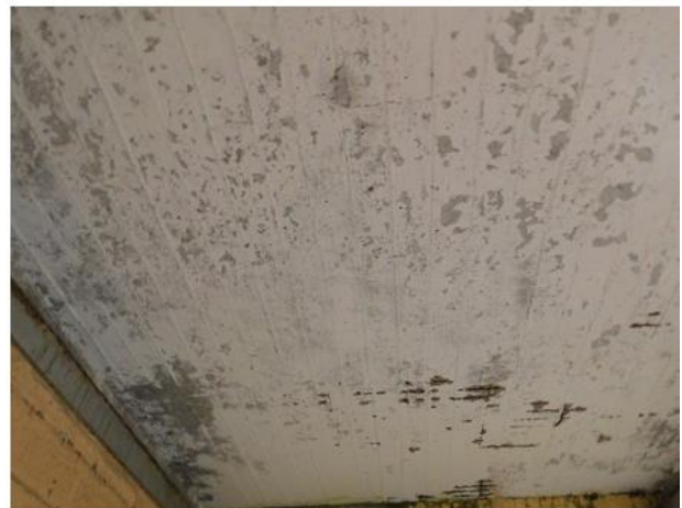
PHOTO 28 Underside of Building 3 Eastern Roof
