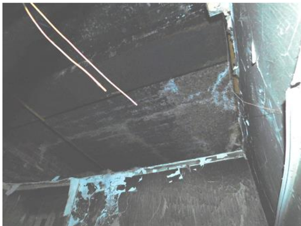
PHOTO 23 Underside of Building 2 South-western Roof
