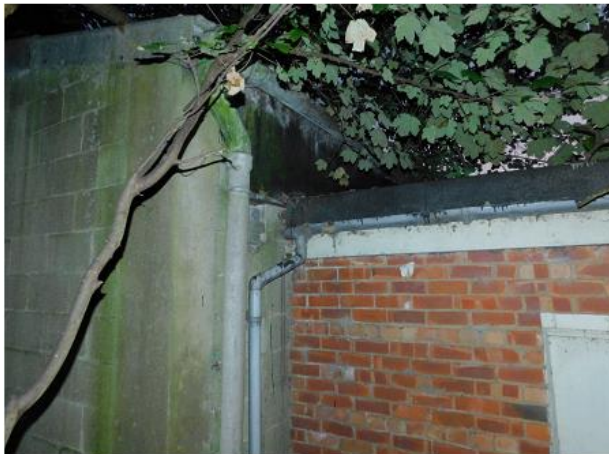
PHOTO 17 Junction of Buildings 3 and 4
