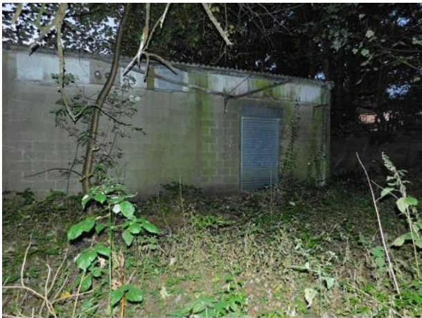
PHOTO 13 South-eastern Elevation of Building 4
