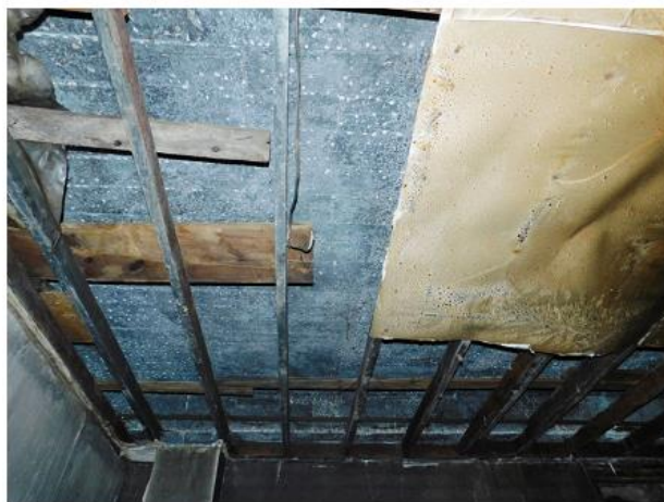
PHOTO 22 Underside of Building 1 Roof
