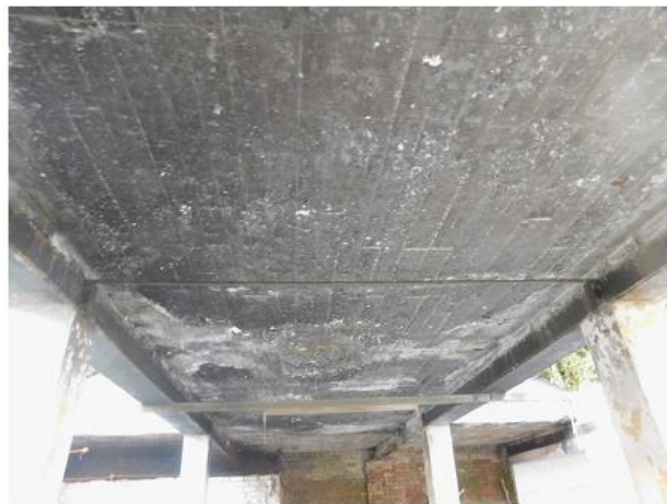
PHOTO 24 Underside of Building 2 Northern Roof
