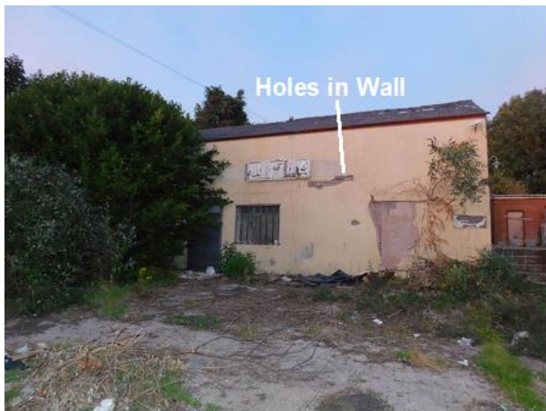
PHOTO 1 Western Elevation of Building 1
