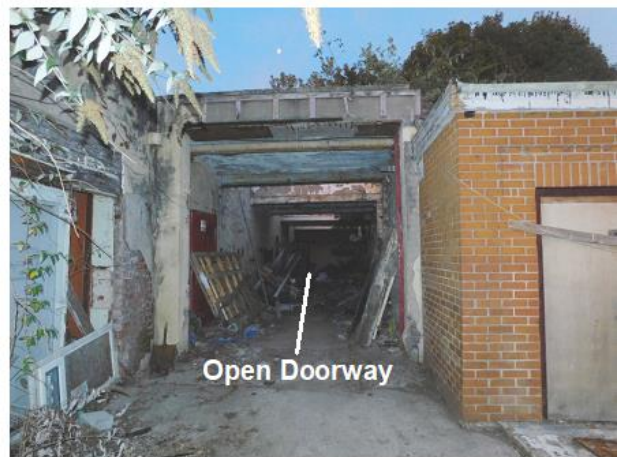
PHOTO 6 View along Southern Elevation of Building 2
