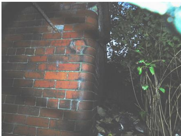
PHOTO 19 South-eastern Corner of Building 2
