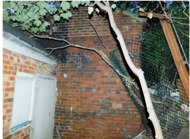
PHOTO 18 Junction of Buildings 2 and 3
