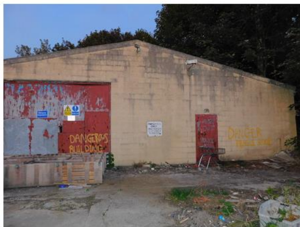
PHOTO 10 Western Elevation of Building 4
