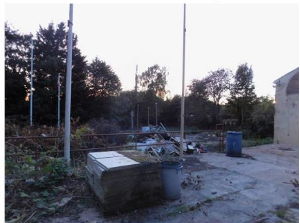
PHOTO 4 Western View across Concrete Hardstanding
