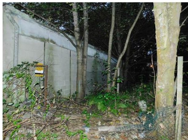
PHOTO 11 South-western Corner of Building 4
