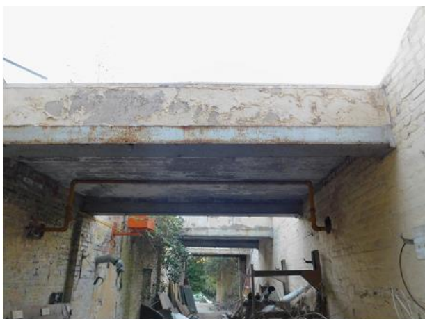
PHOTO 7 View Along Building 2 Passageway
