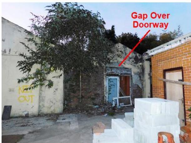
PHOTO 5 South-western Corner of Building 2
