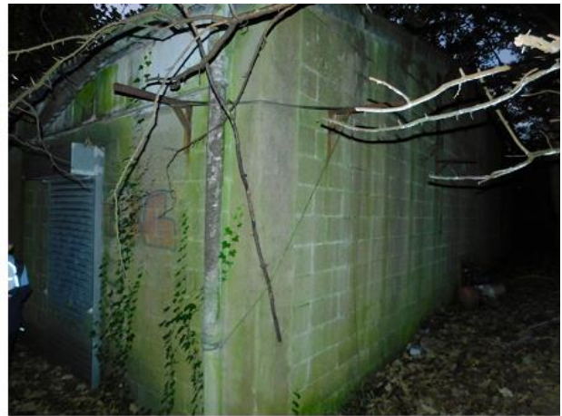
PHOTO 14 South-eastern Corner of Building 4
