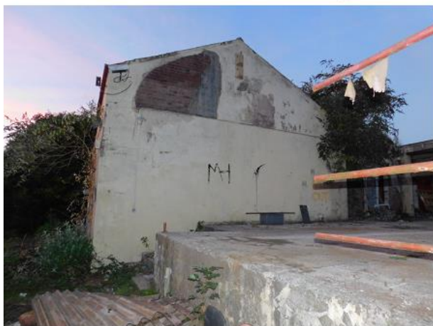
PHOTO 3 Southern Elevation of Building 1
