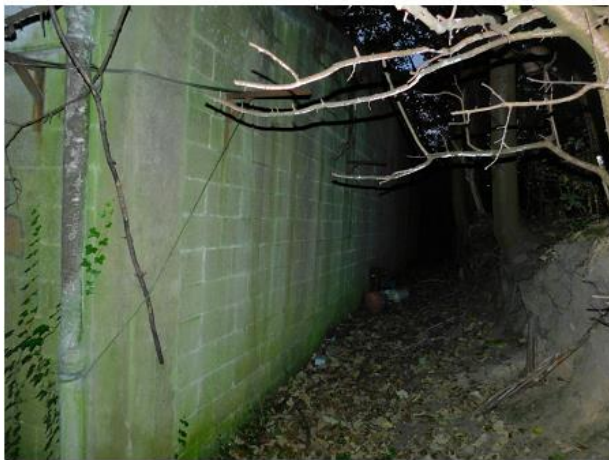
PHOTO 15 View along Eastern Elevation of Building 4
