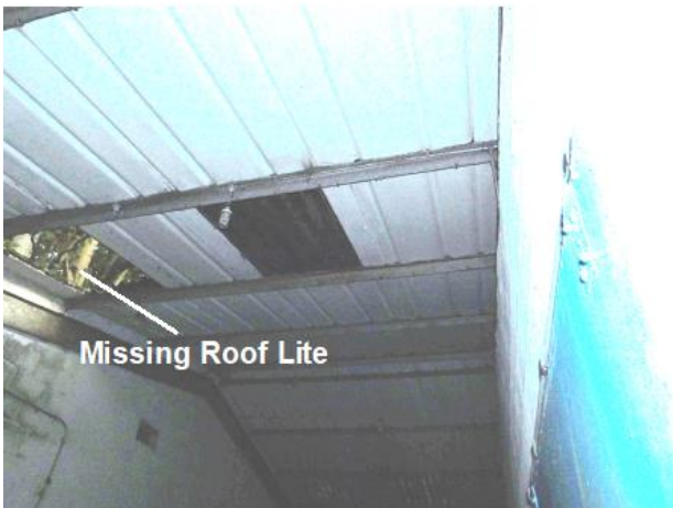
PHOTO 29 Underside of Central Roof of Building 4
