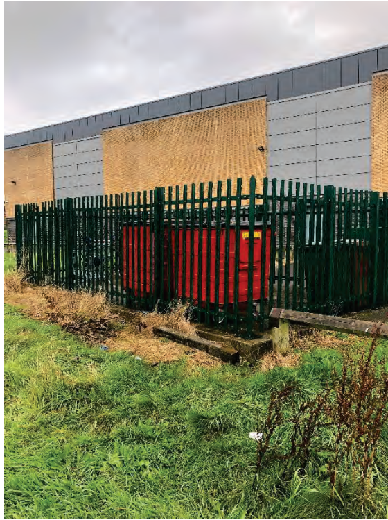
Photo 12: Fenced off bin storage
