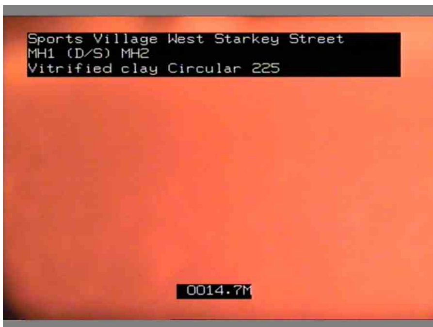
_20b8fcea-598f-4eca-b584-d5b15450e5db.jpg, 00:01:34, 14.60 m Camera under water, Start
