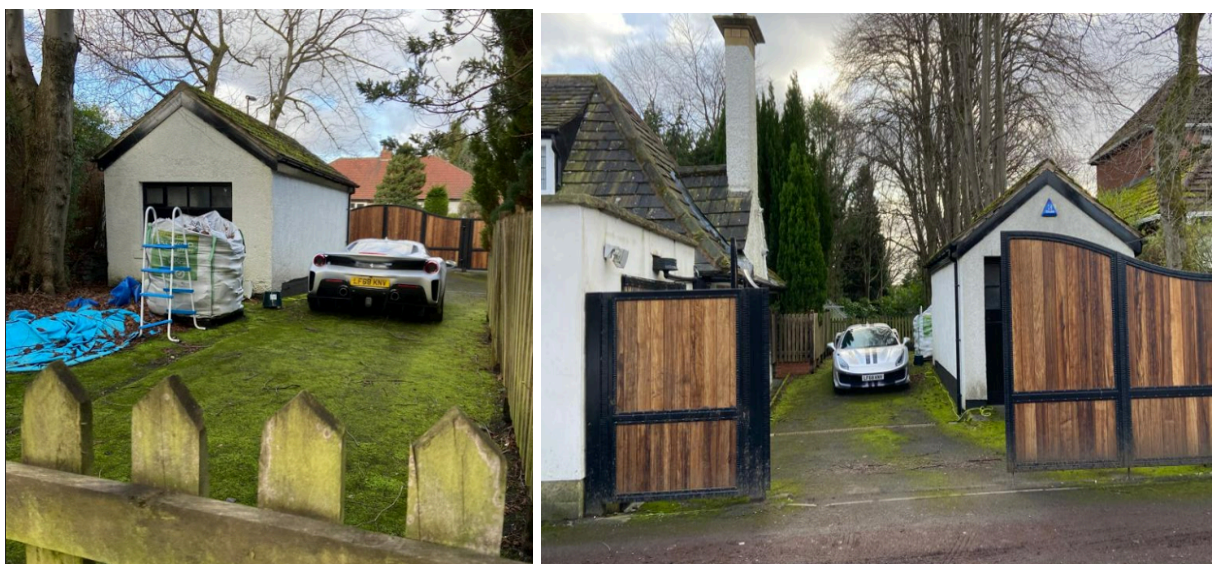
Figure 1 Rear view of the existing building and view from the road.
